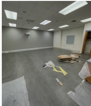
Rowe Lane Elementary Classroom Progress
