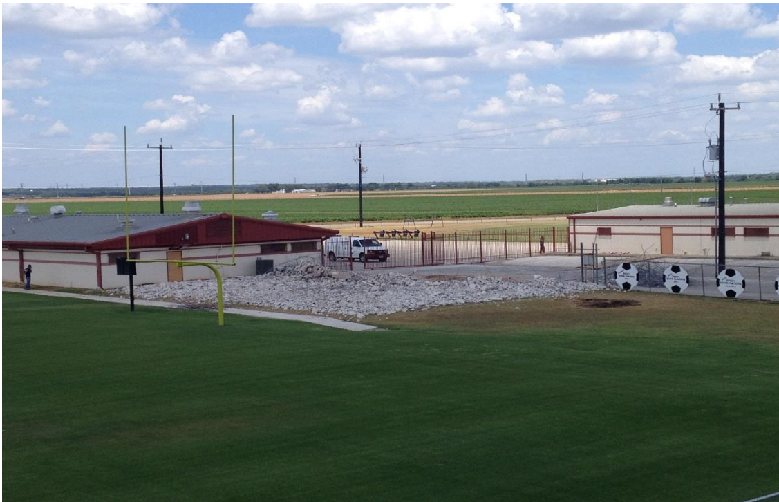
East End of Stadium (Demolition of old Field House slab)
