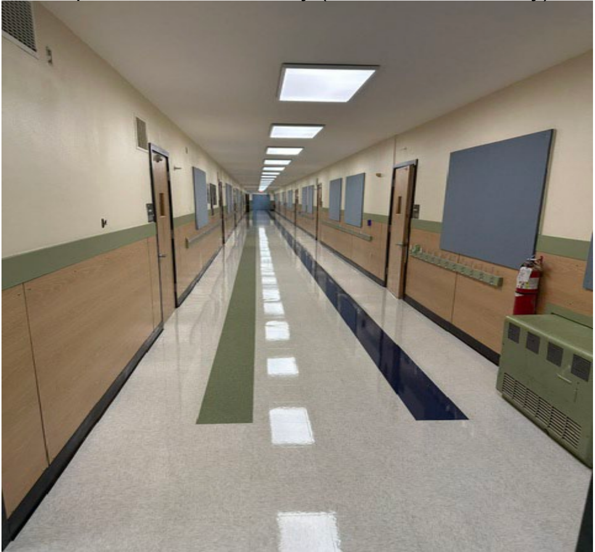
Yaquina View Elementary (construction hallway)
