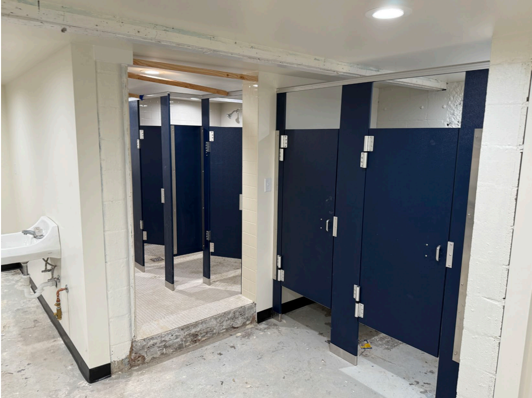
Locker room painting was completed and new toilet & shower partitions were installed.
