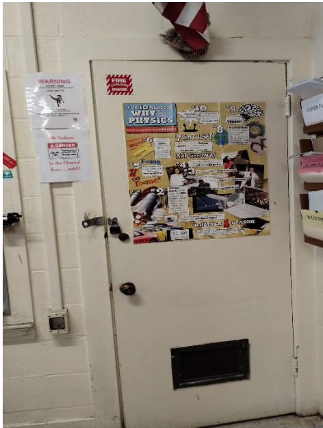
Chemical storage in chem lab. Ensure chemical storage area is prominently signed and secured at all times.
