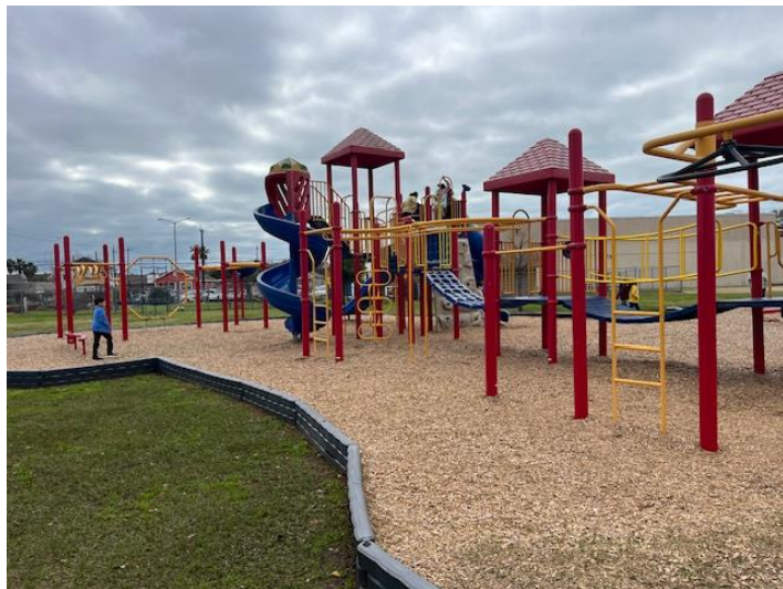
playstructure #4 Climbing structure is combines in large playground – this needs 25' x 25' area
