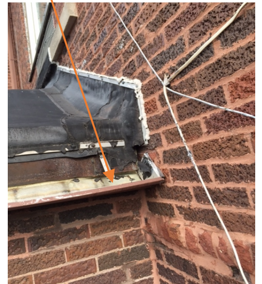
Gutter Damage
