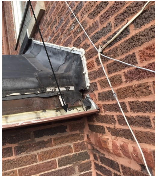
Gutter Damage
