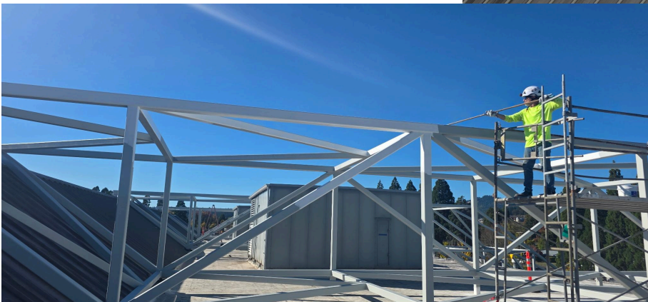
Painting the steel exoskeleton
