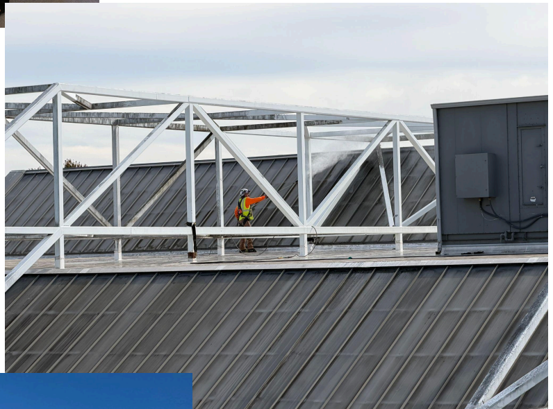
Power washing the roof in preparation for paint on the exoskeleton
