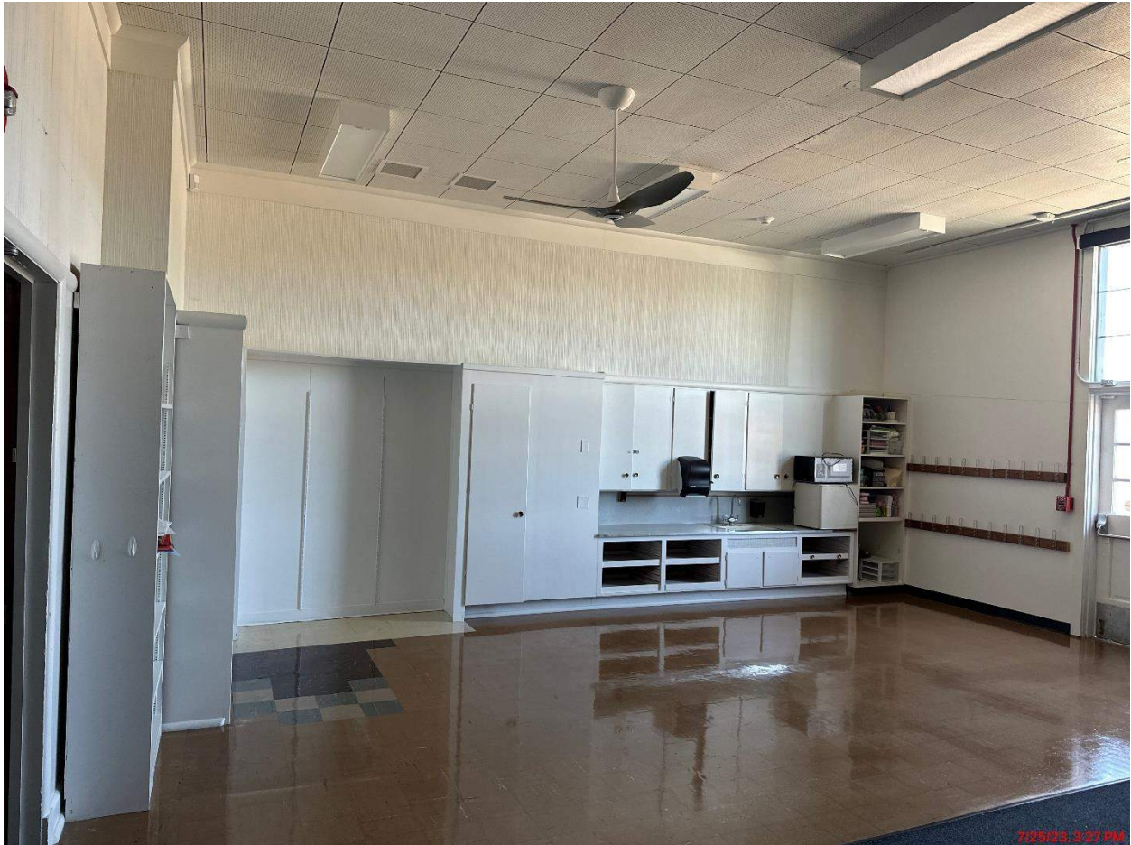
Franklin – New Classroom painted walls and ceilings.
