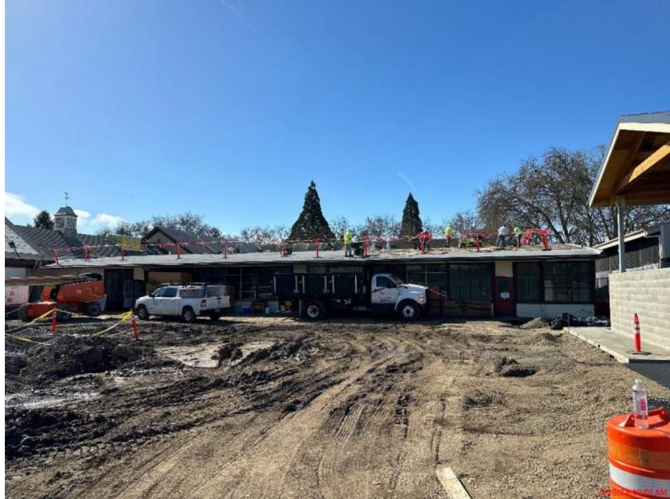
CHHS – B wing re-roofing
