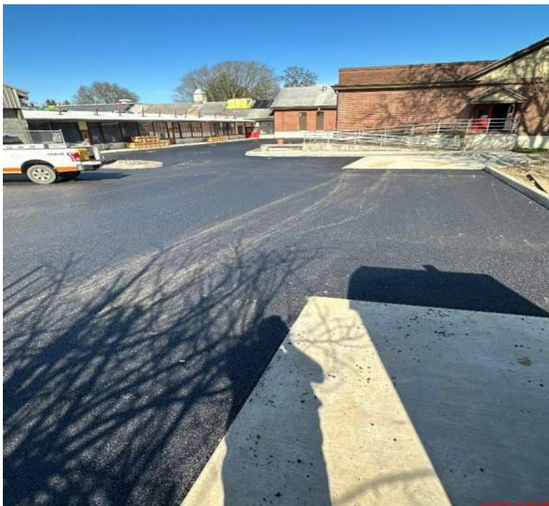
CHHS – New paving between A wing and B wing
