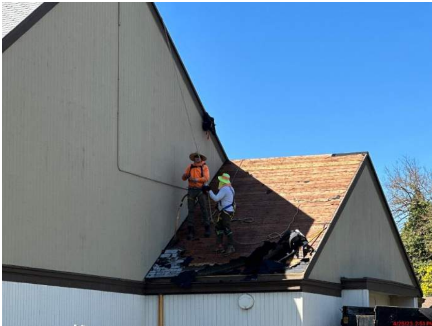
CHHS – Re-roofing Gym
