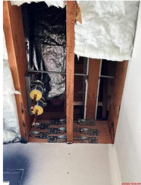
CHHS – some of our final evidence of new seismic work
