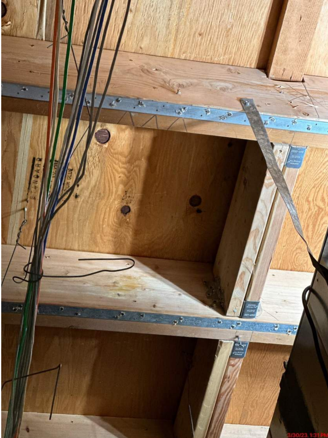
Cheldelin - Duct penetration reinforcement
