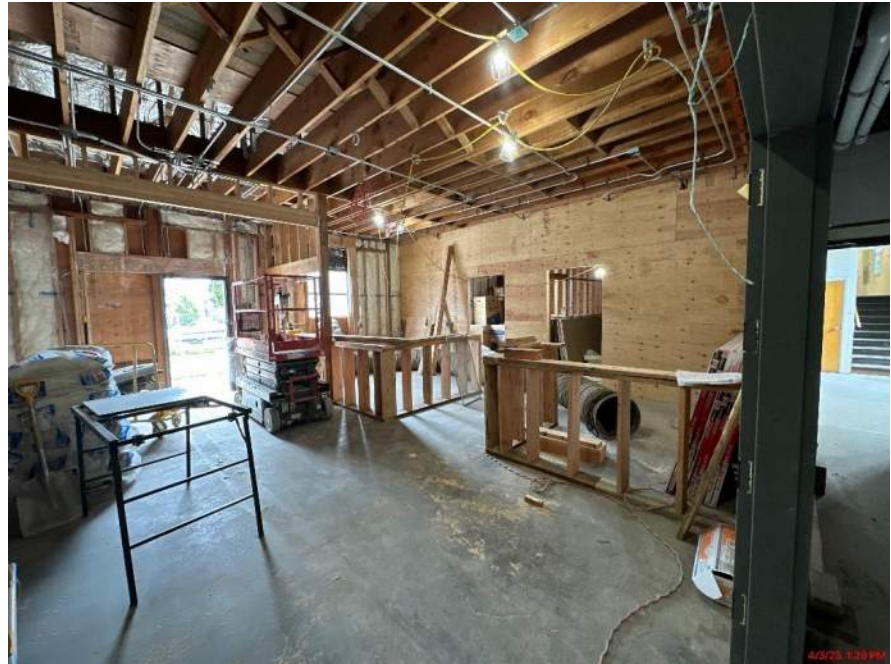
CHHS – Front office walls taking shape
