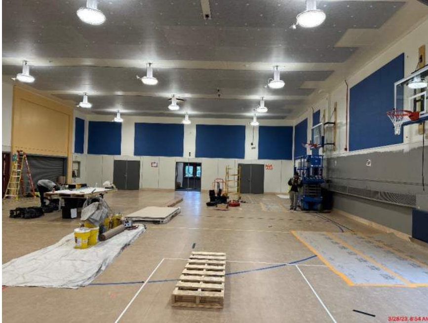
Franklin – Gym acoustical panels and FRL installing
