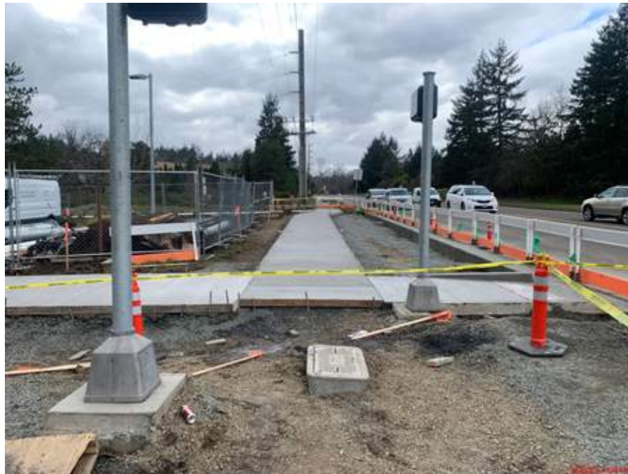
Aspen intersection work
