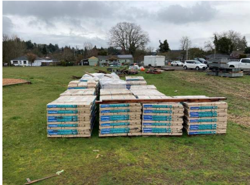
CHHS – Roof shingles onsite and ready for install
