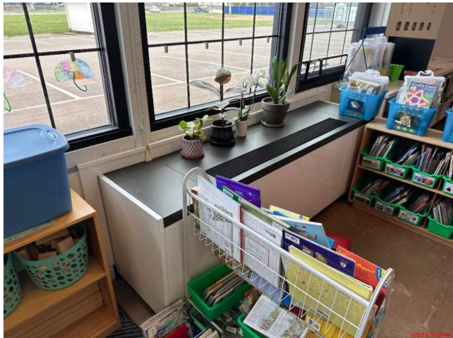
Franklin – New unit ventilator in place
