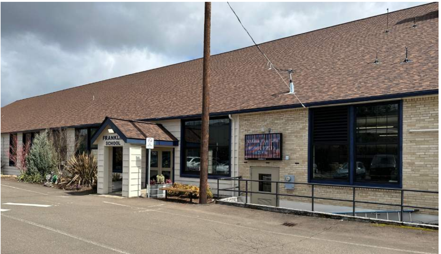
Franklin looking good, with a new roof, new windows, new reader board and new paint!
