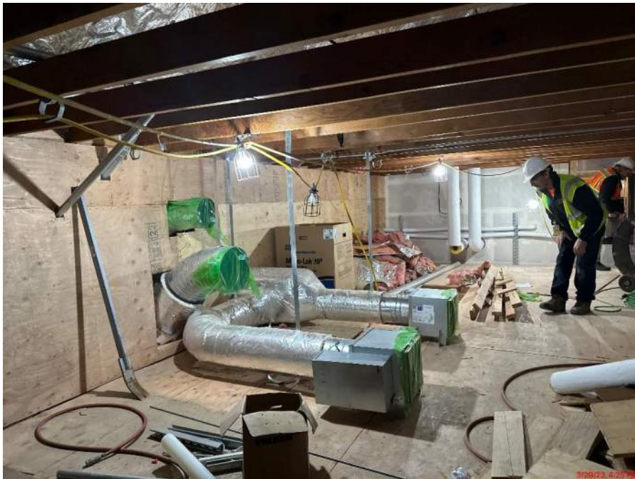
CHHS – misc. ductwork installation in attic space
