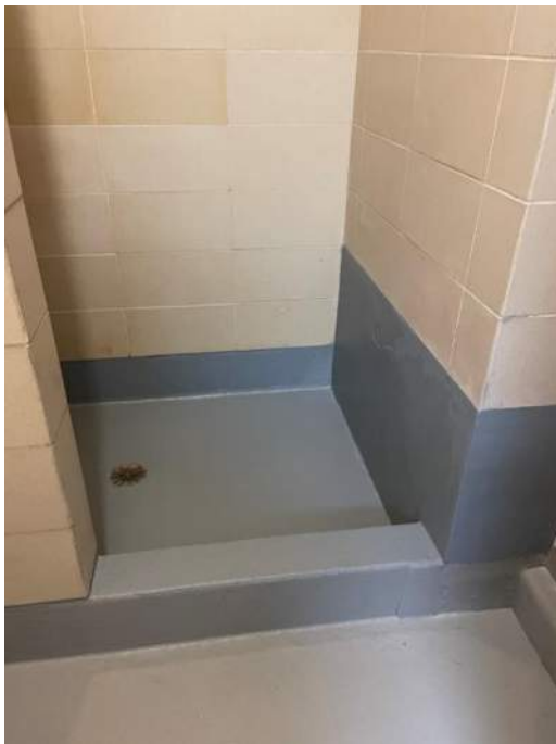
CMS – Shower repairs completed
