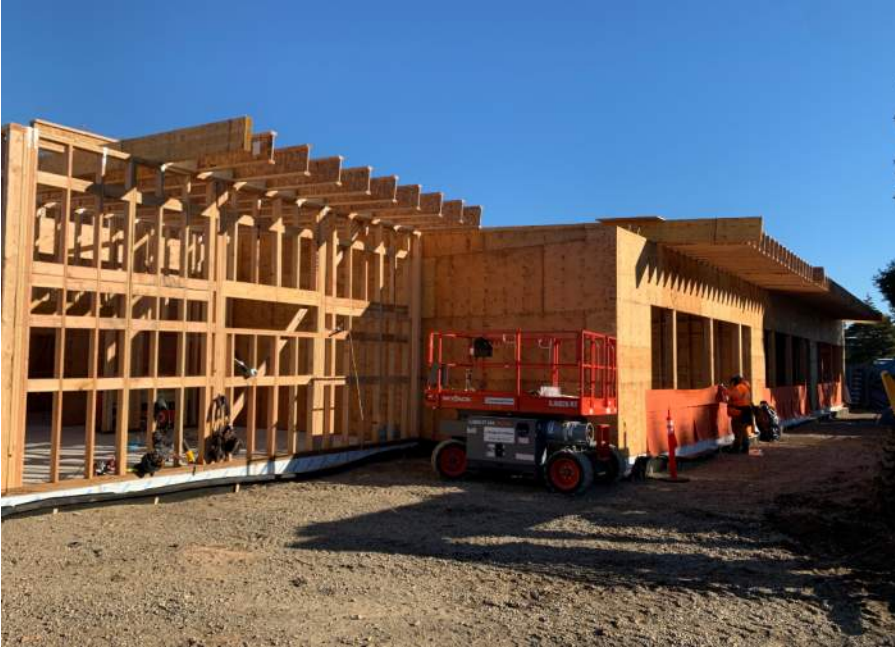
New Classroom Wing Framing
