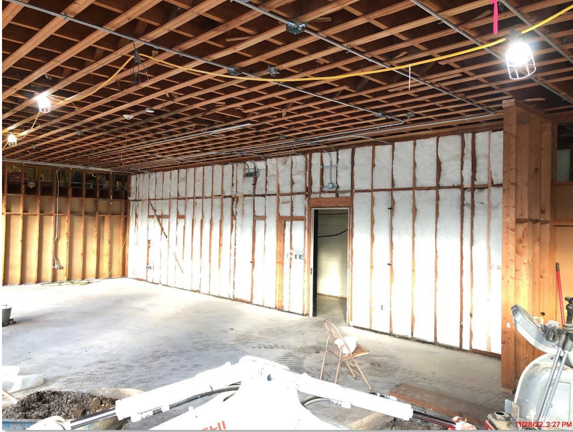
Sound Insulation Installed on Classroom Corridor Wall
