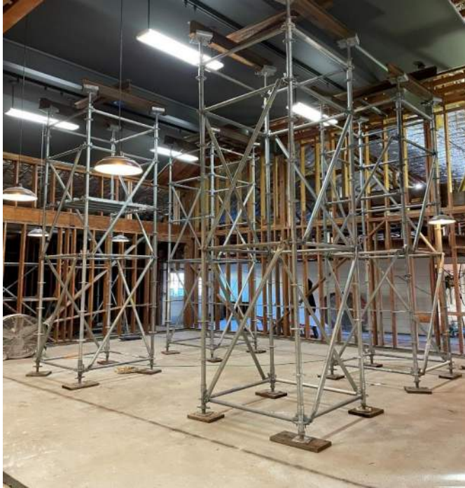
CHHS – temp shoring for reframing efforts
