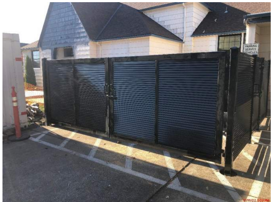
Trash enclosure finished
