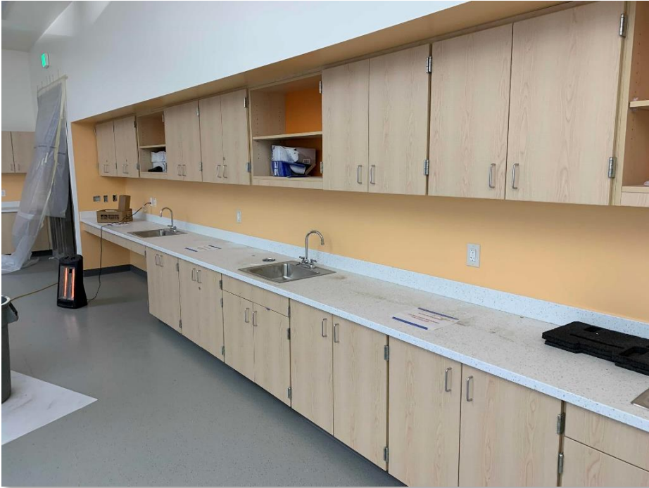
Science Classroom Progress
