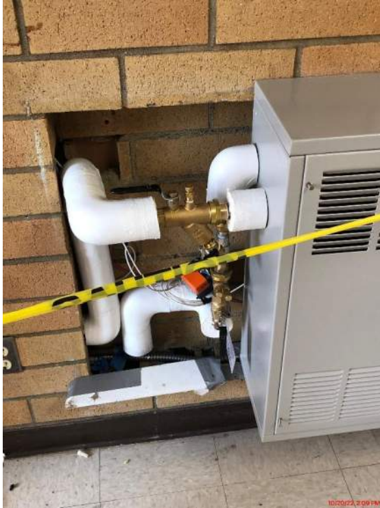
CMS – Cabinet Unit Heater Installation
