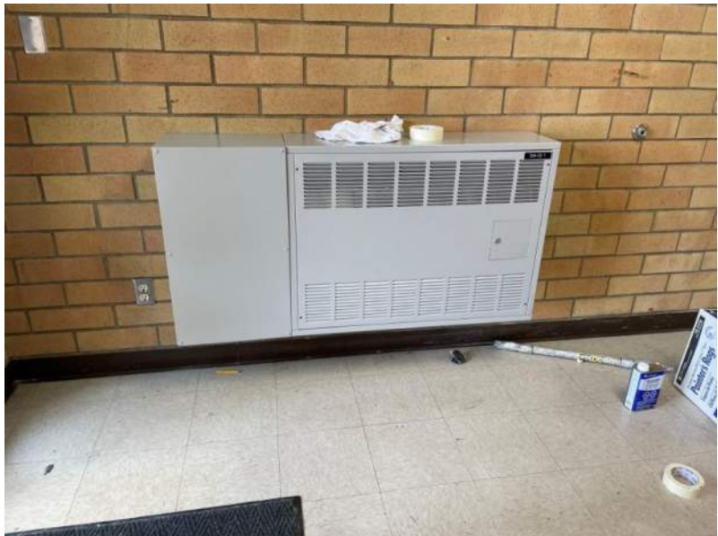
CMS – Cabinet Unit Heater Installation
