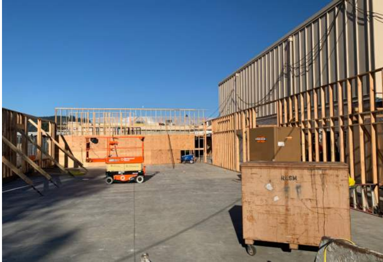
Art / Science Wing wall framing
