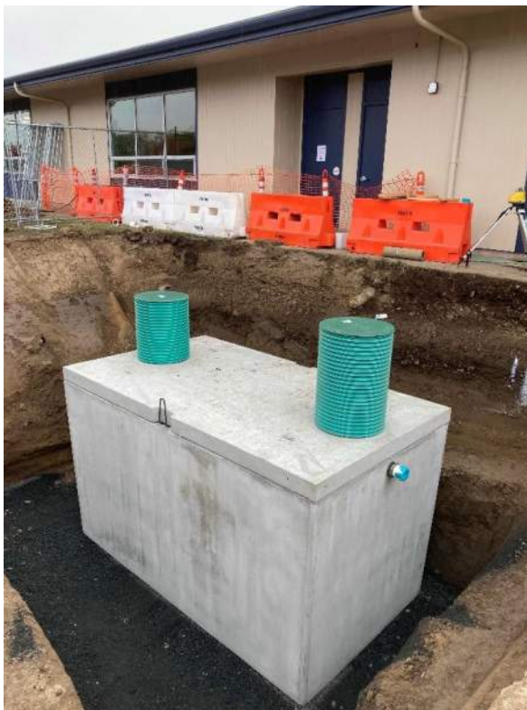
Installation of new septic tank
