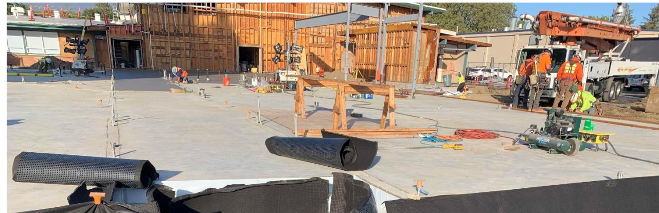
New Addition Slab
