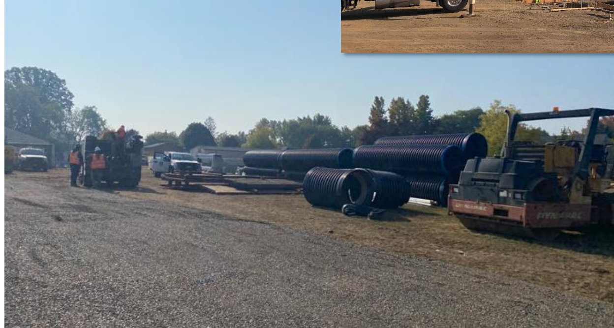
Storm Piping Staged
