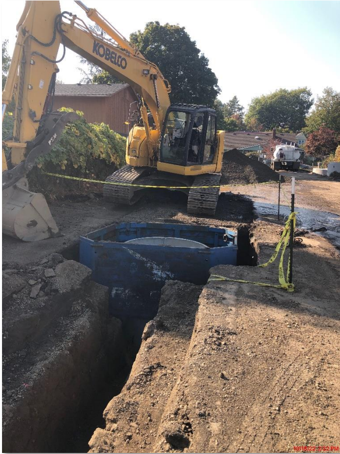
New On-Site Storm Manhole
