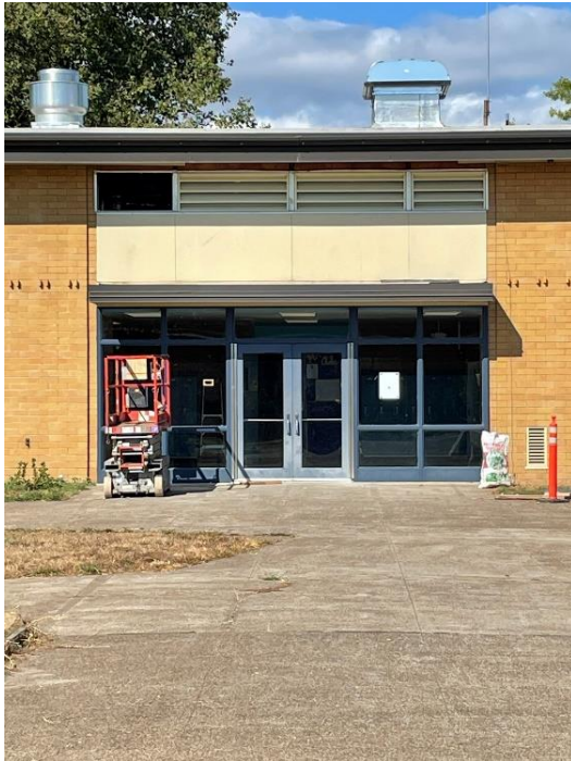
CMS – Louver Installation
