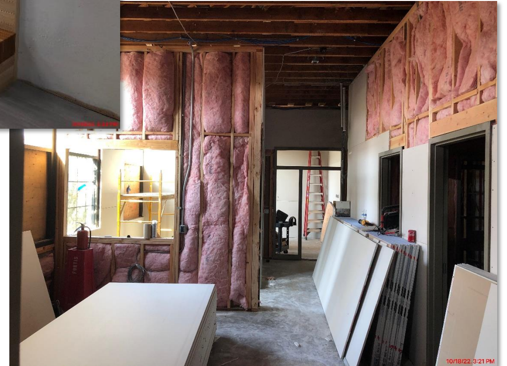
New Admin Space Progress
