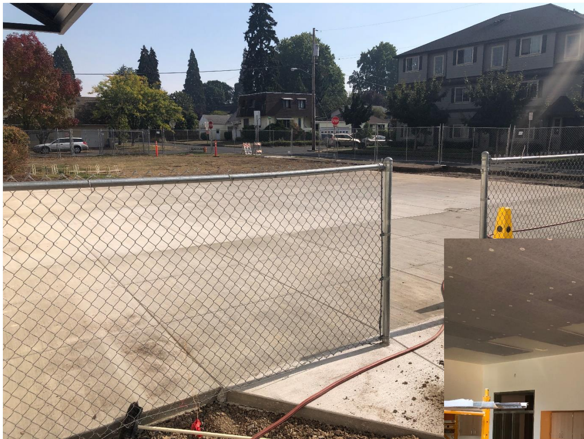
New Patio Has Been Placed
