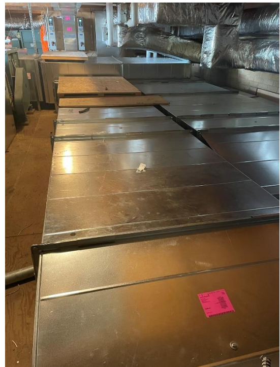
CMS – New Larger Ductwork Sections
