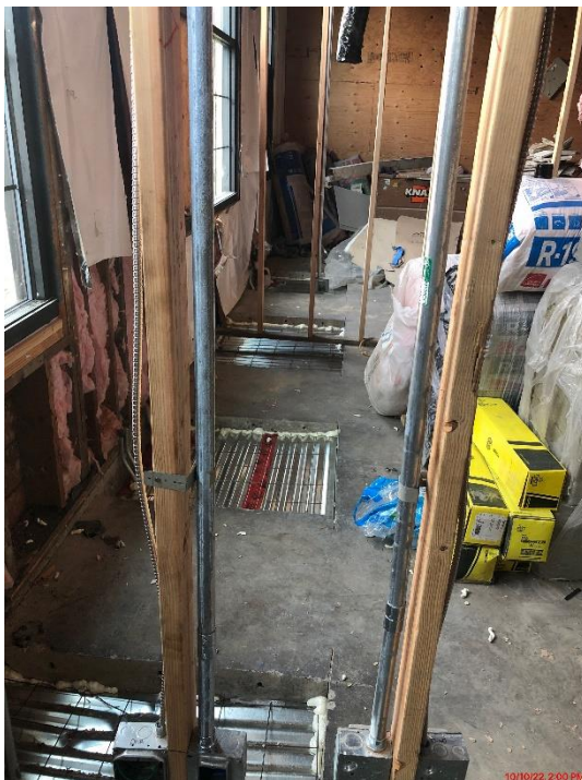
New Admin Tunnels Prepped for Slab Pourback
