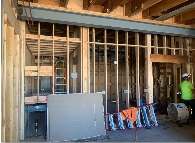
Admin Renovation Underway
