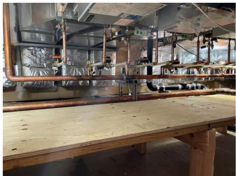
CMS – mechanical replacement progress
