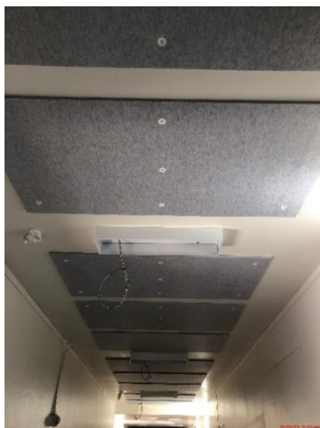
Franklin – new corridor acoustical panels
