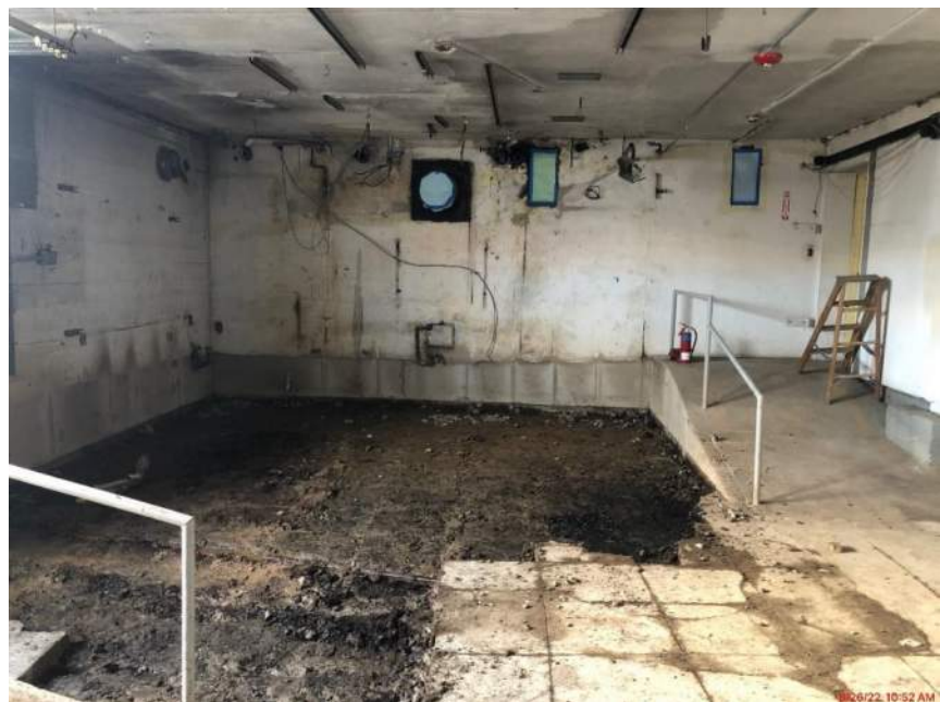
College Hill – Boiler Room Demo
