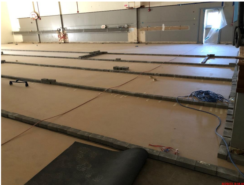
Gym Flooring in place, with protection still in place. Bricks are used to help seal the joints in the material.
