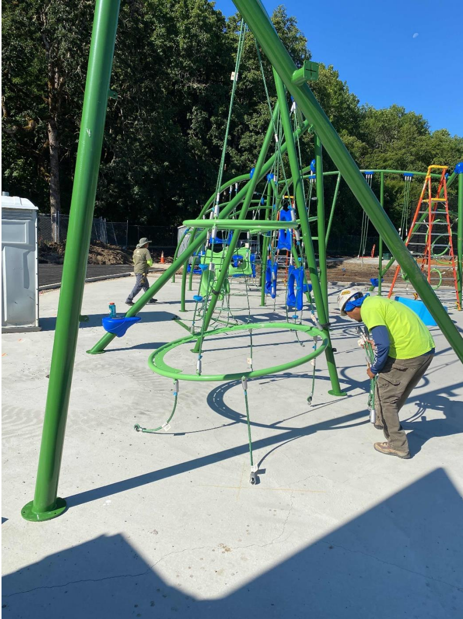
Playground Installed - Awaiting Play Tile Crews
