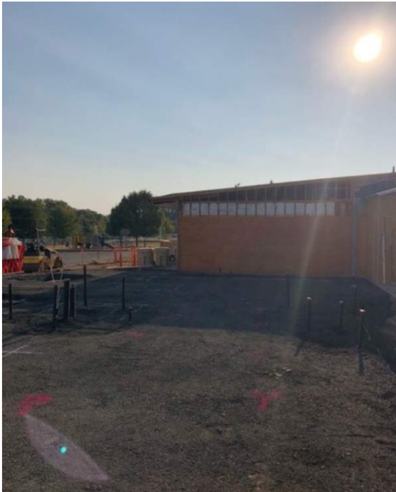
Admin Suite underground work
