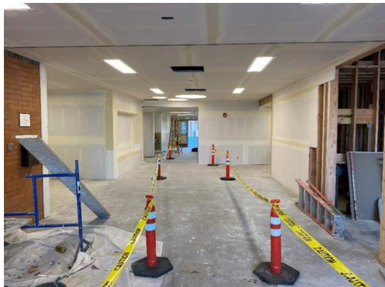
Main Entrance Lobby
