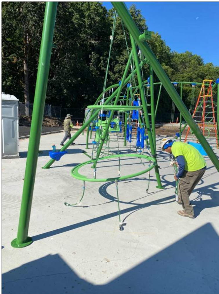
Almost ready for safety play tile
