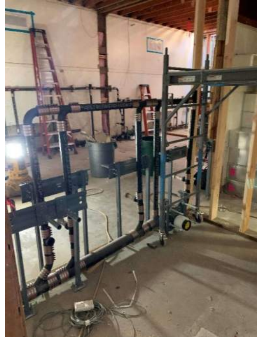
New plumbing rough-in
