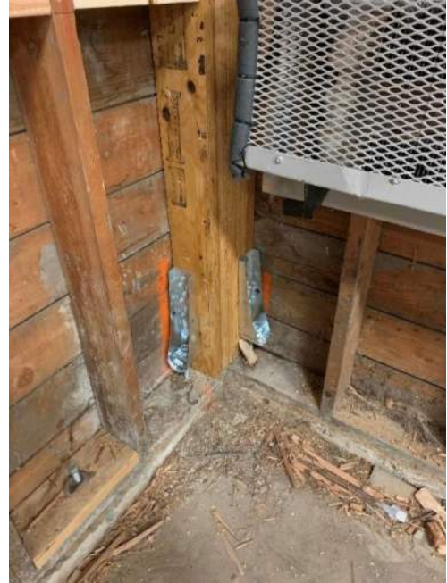
New seismic hold downs in existing walls
