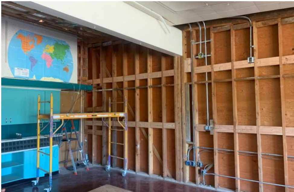
Classroom seismic blocking and technology rough-in
