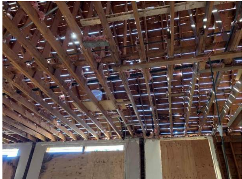
Office Ceiling demo progress
