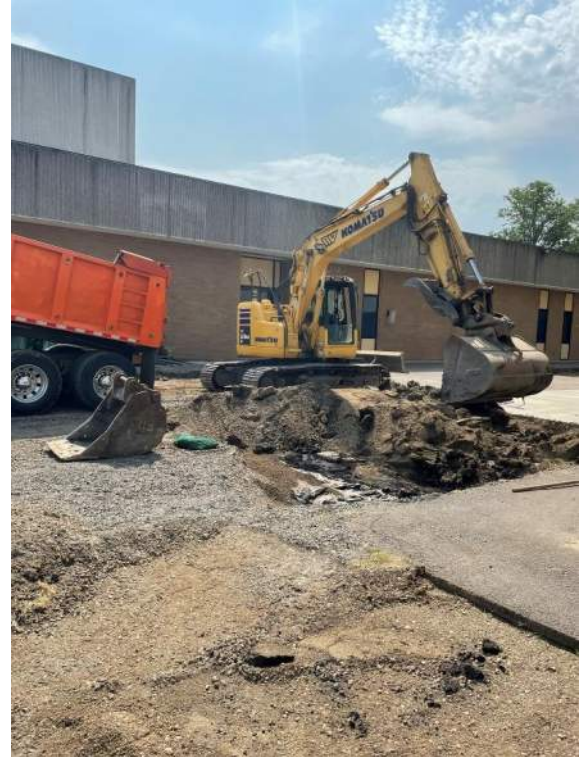
Cleanup between Bldg. A & B
