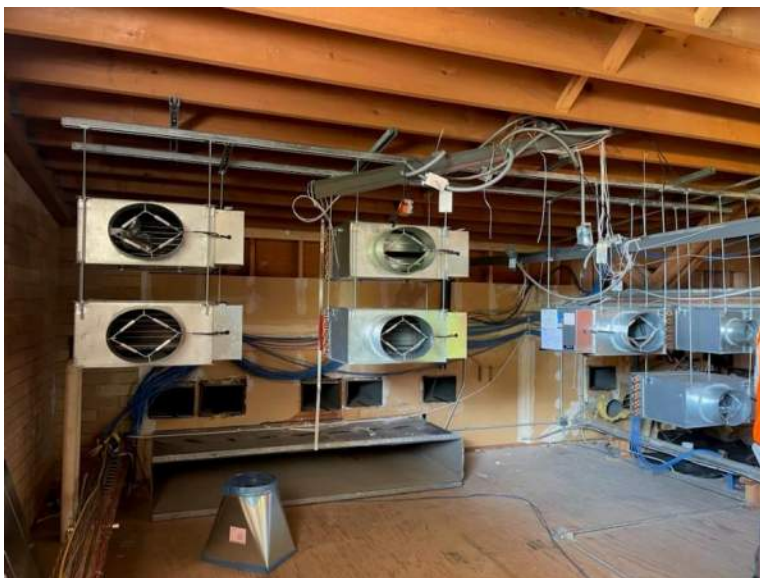
CMS – Classroom wing mechanical room HVAC rebuild
