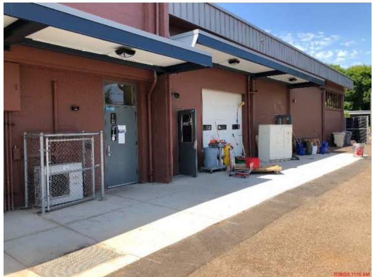
AT south canopies complete
