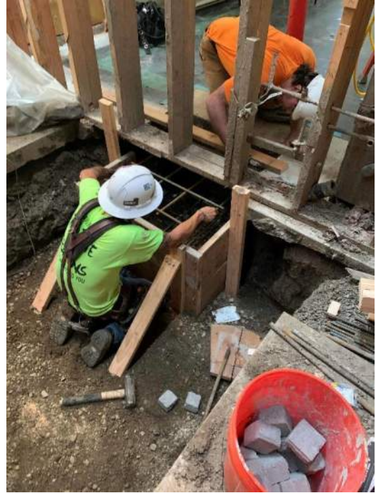
New interior footing work
