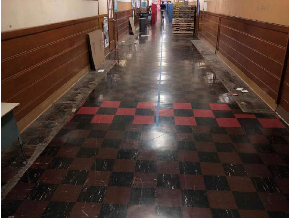
Franklin hallway after locker removal
