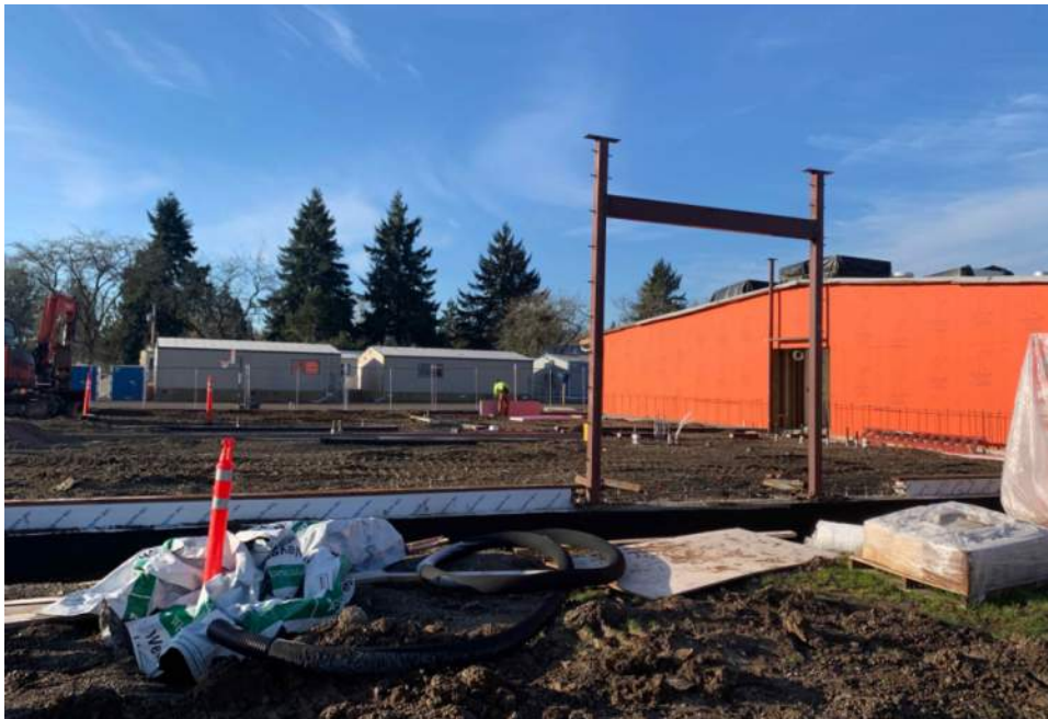
Slab Prep at Classroom Addition
