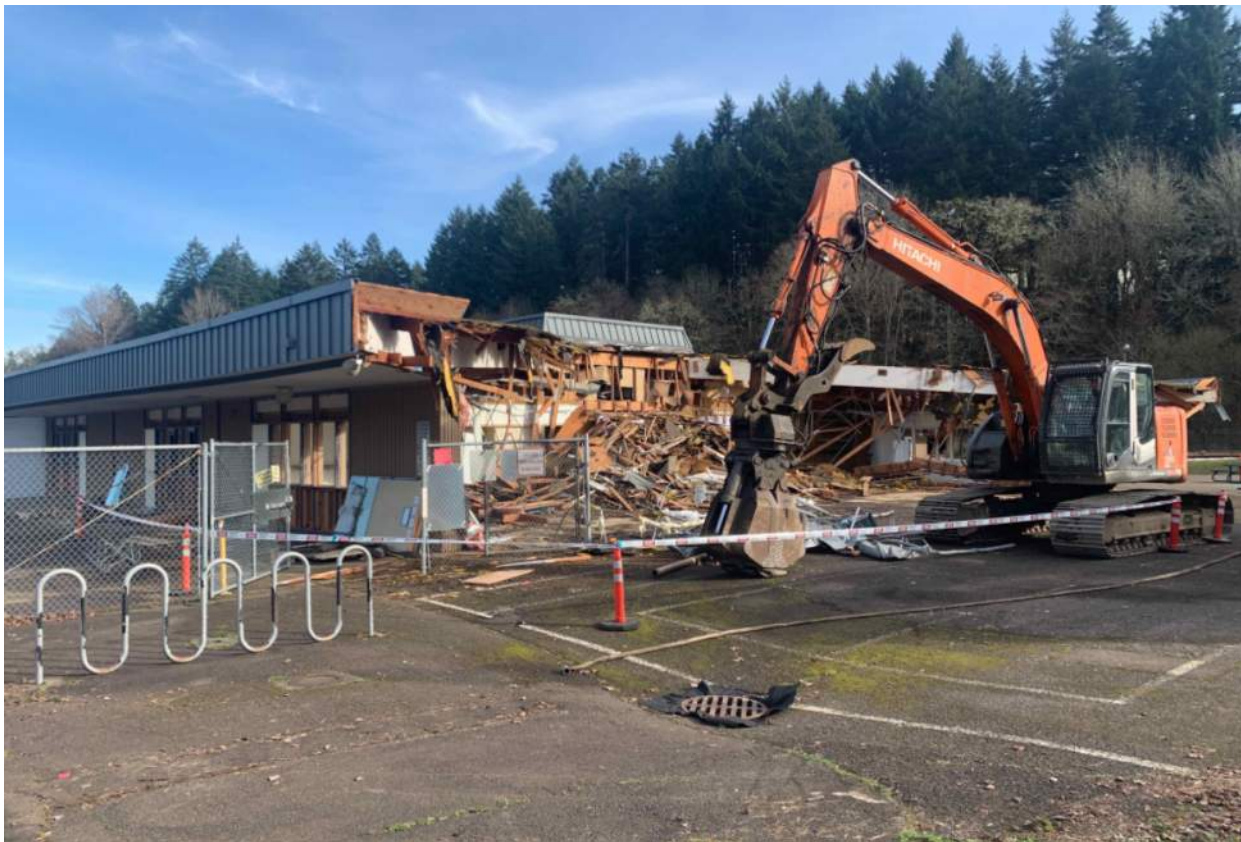
Demolition of Old Structure
