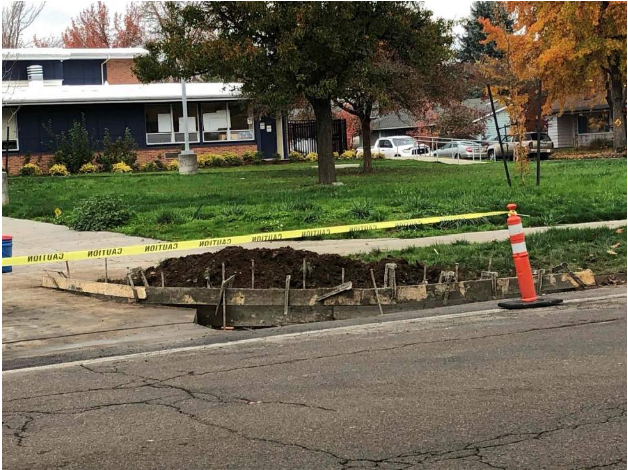
Final construction for driveway approach
