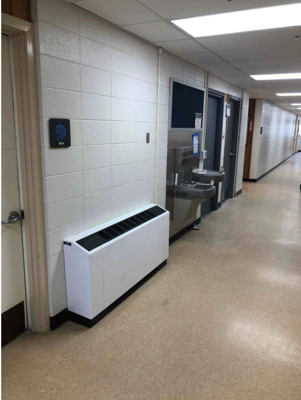
CHS – AT North – Hollow metal doors and drinking fountains installed
