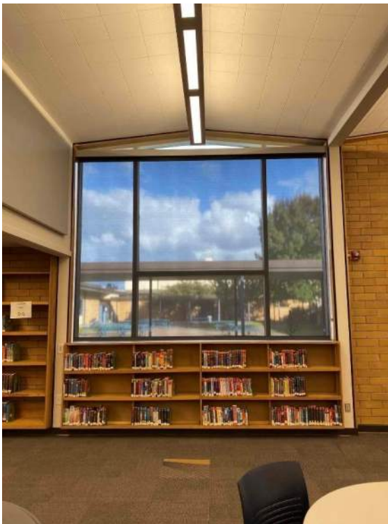
CMS – new library roller shade installed
