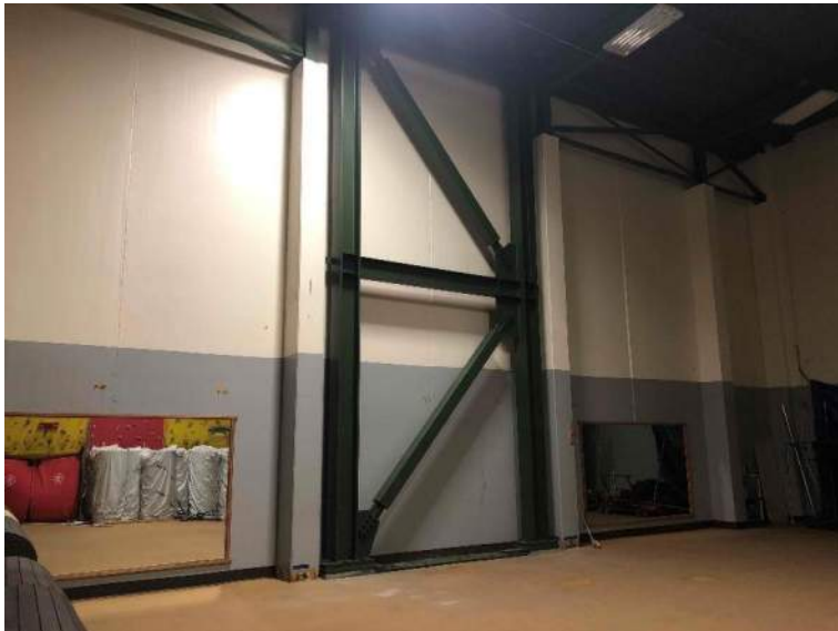
CVHS – Building A - gymnastics seismic frame 100%
