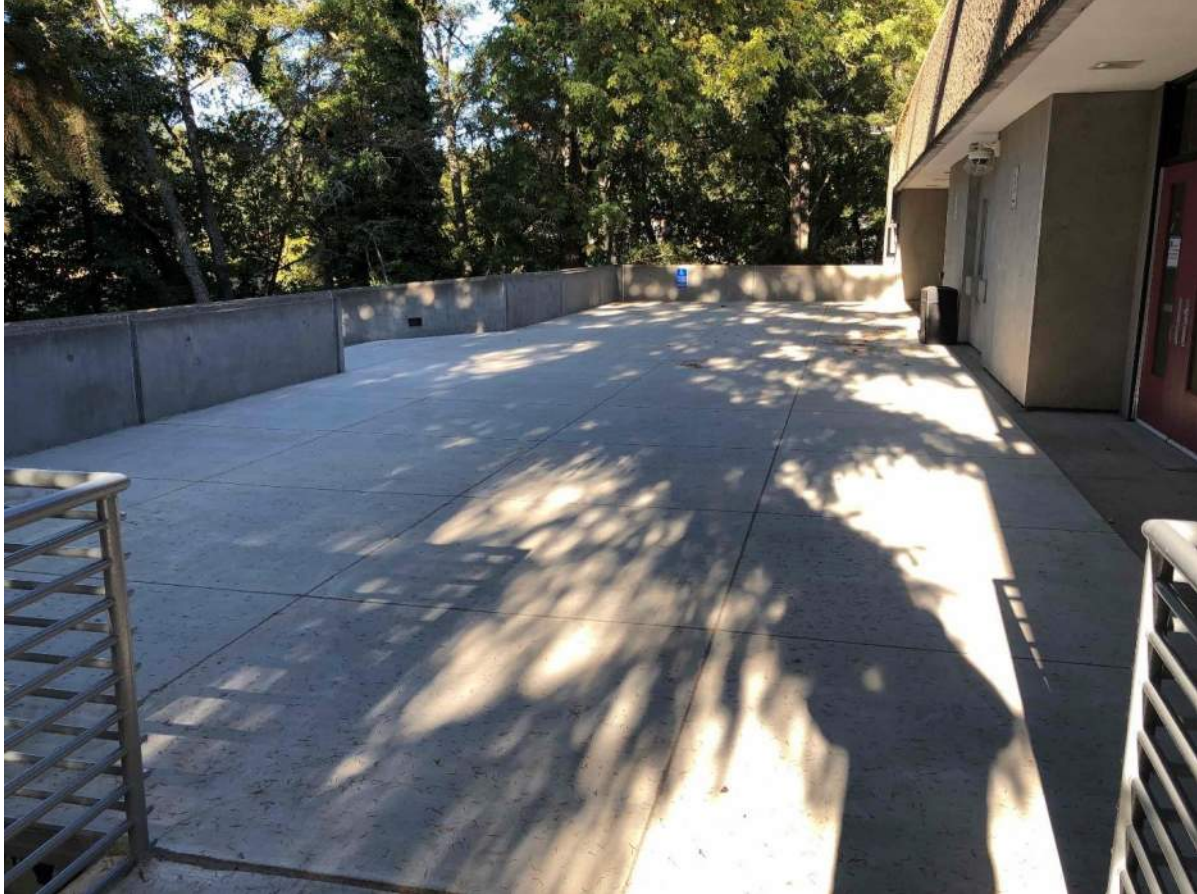
CVHS Building A – Topping slab finished and sealed
