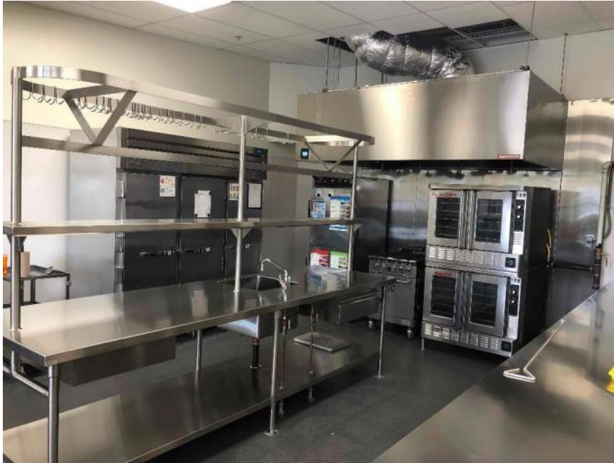
Garfield - New Kitchen Hood and prep island – ready to move in
