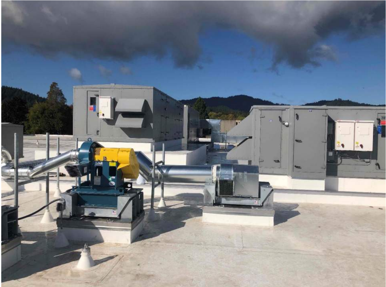
CVHS – Building F - New HVAC units and exhaust fans 100%
