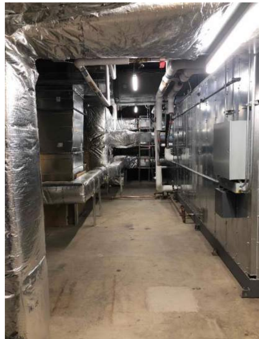
CVHS Building F – New mechanical mezzanine
