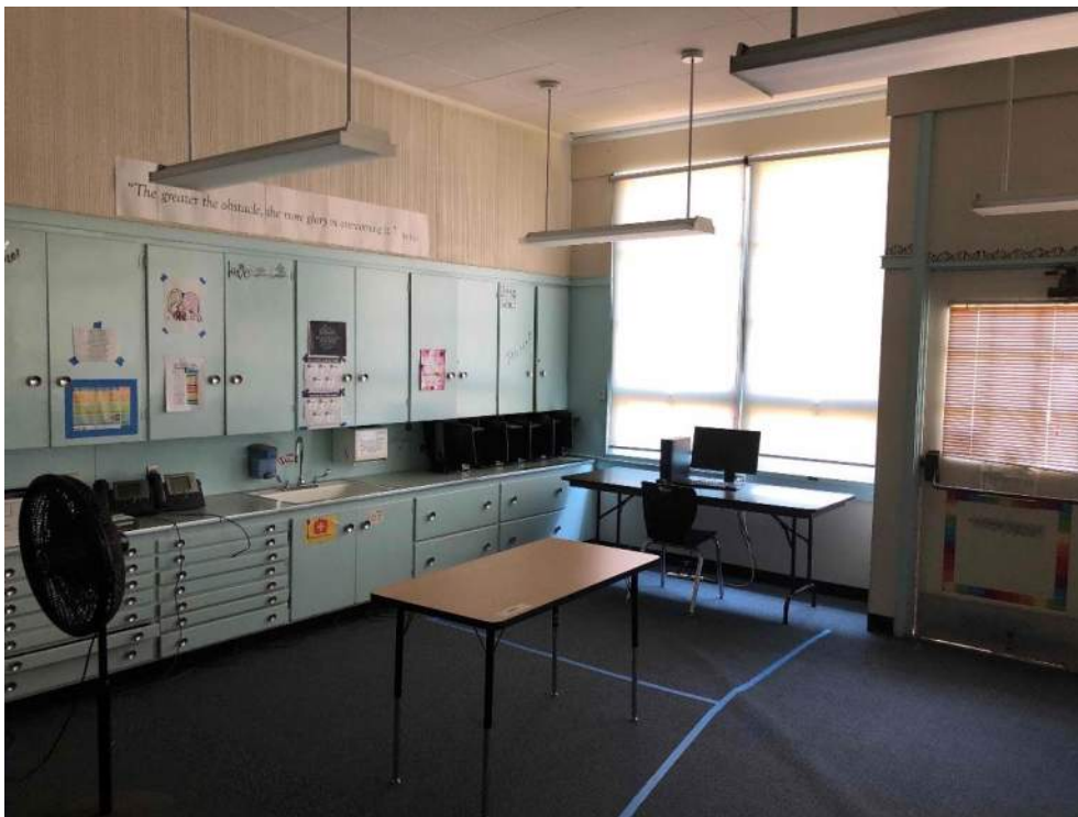
College Hill – Classroom casework scheduled for renovation
