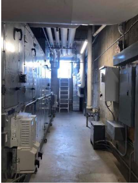
CVHS Building F – New mechanical mezzanine – roof access pathway
