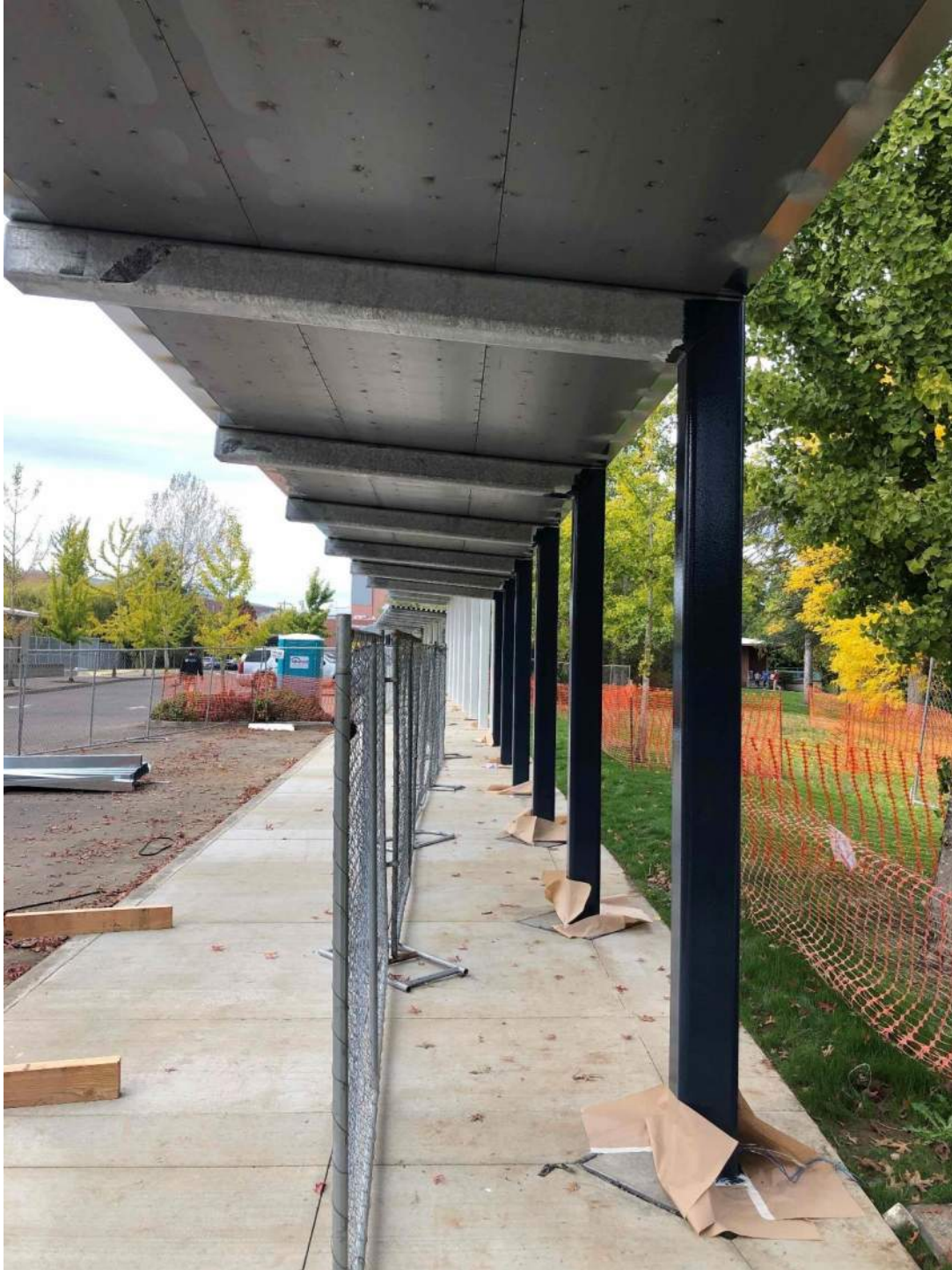
CHS – Covered walkway – decking and painting underway
