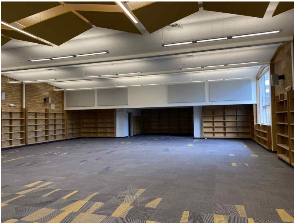
CMS - Front wall & acoustical panels
