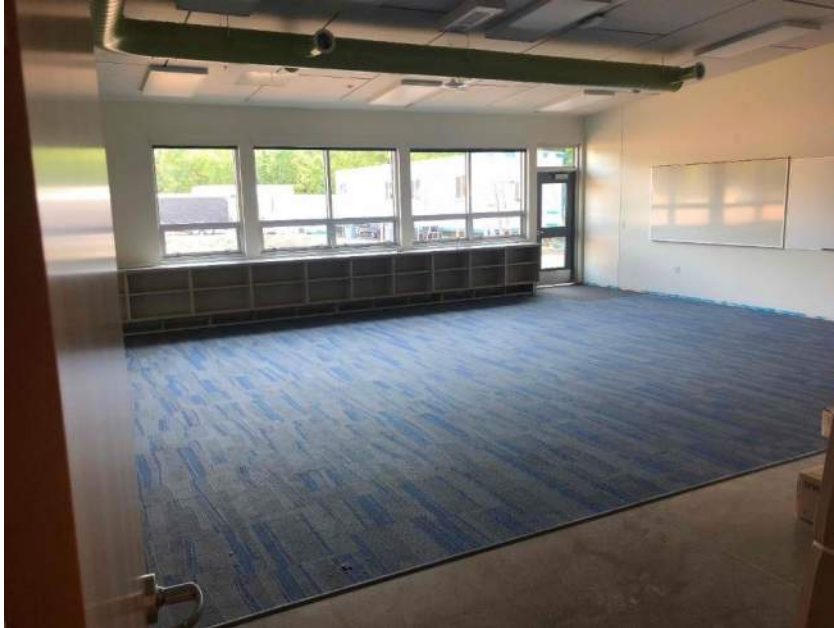
GES – Area C Classroom looking north
