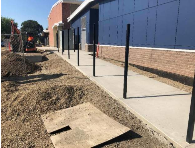
GES – East side ramping and fencing progress
