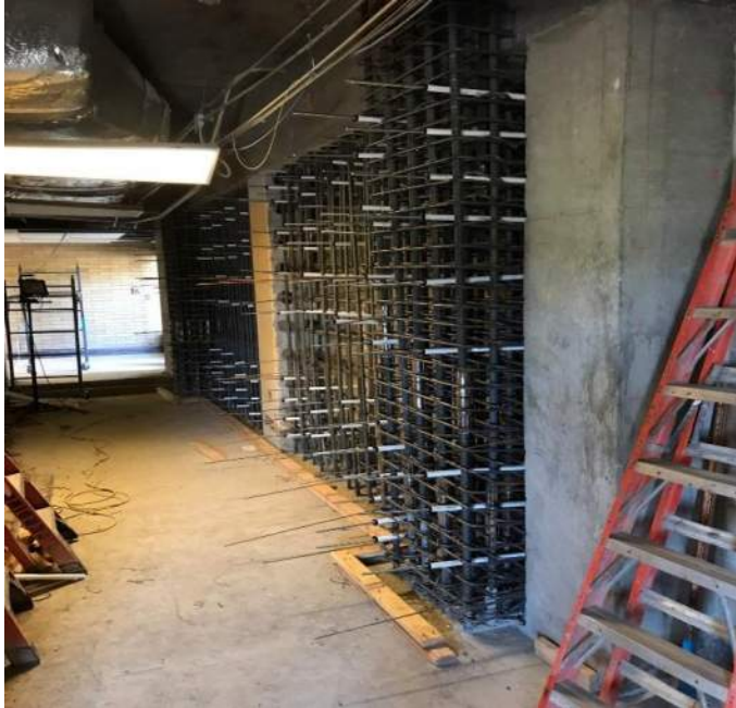
CVHS Building A - Shearwall rebar and formwork
