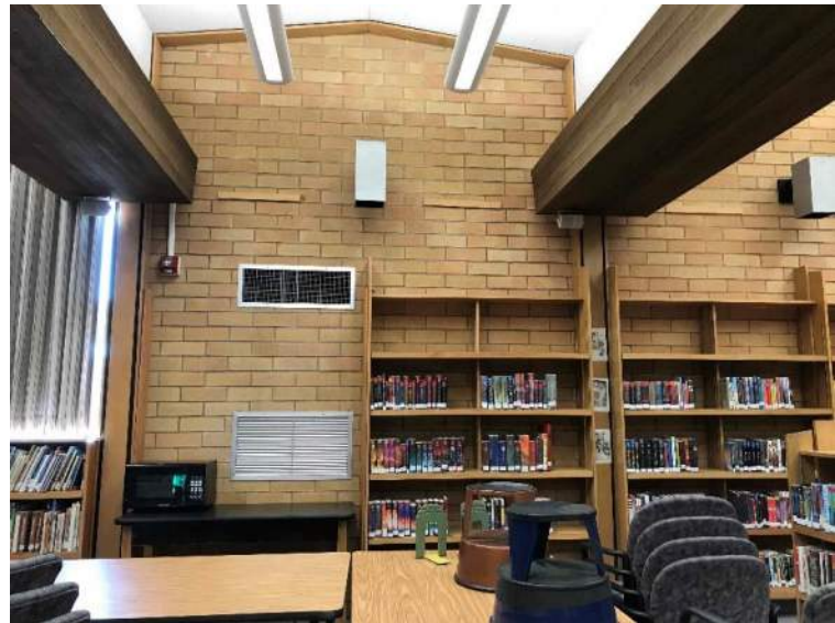
CMS – Previous library ceiling and lighting
