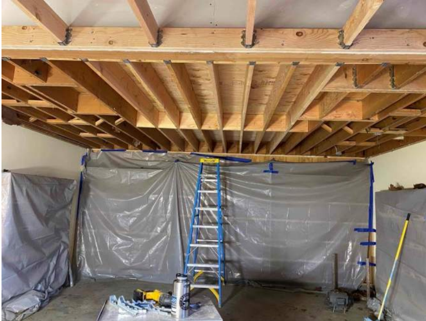
New HVAC mezzanine infill framing
