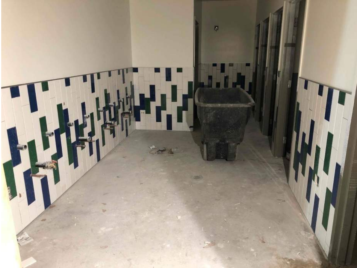
Garfield – Area C new restroom progress
