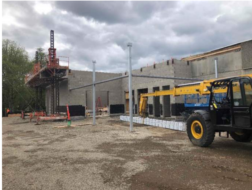
CVHS – New addition and covered work area
