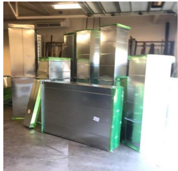
CHS- ductwork staged onsite
