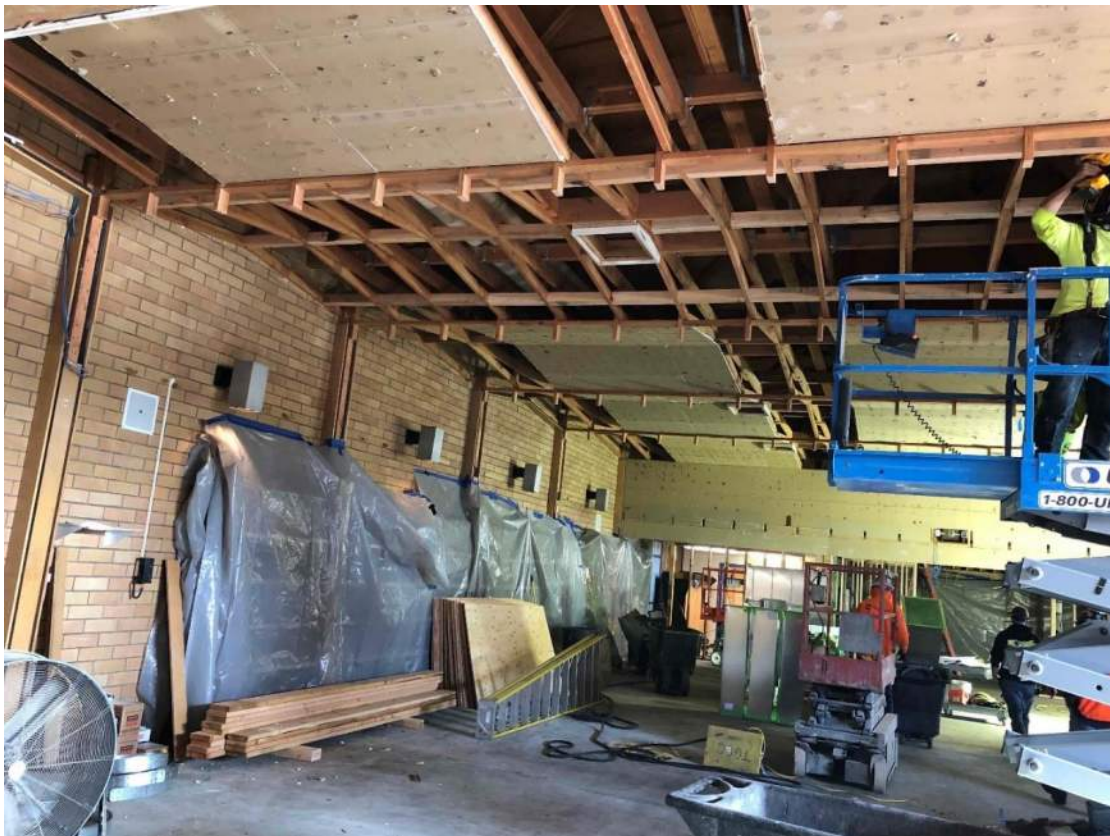
Library ceilings removed in order to remove old duct and to install new ceilings & lighting
