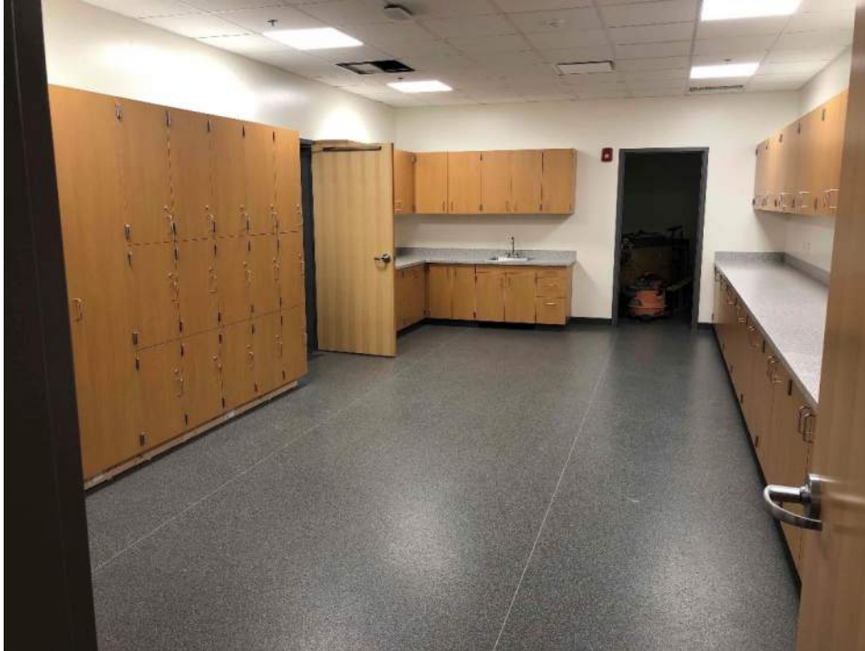
Staff work room - casework done
