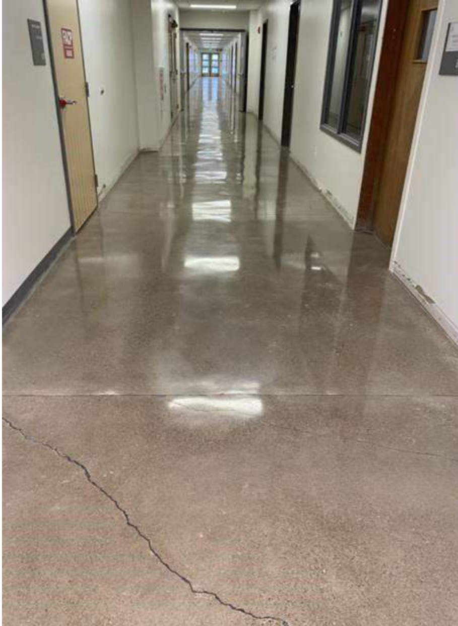
Garfield – Existing concrete, now polished and sealed
