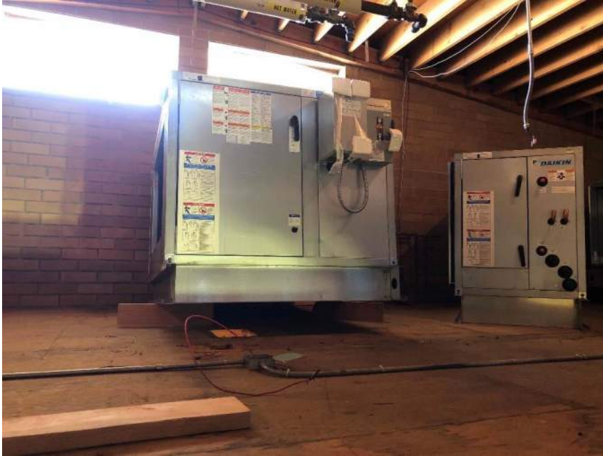
New HVAC installing at north mechanical mezzanine
