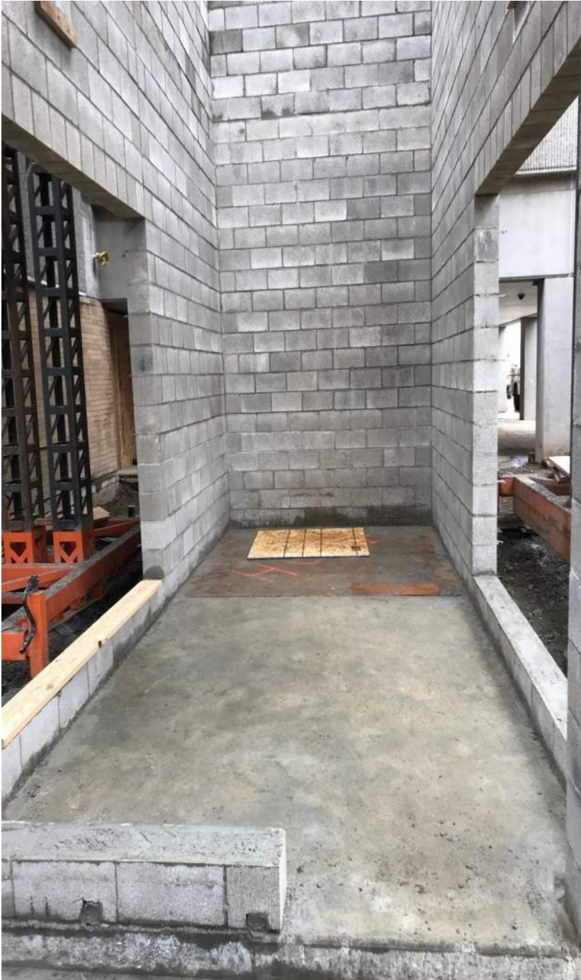
CVHS new elevator walls
