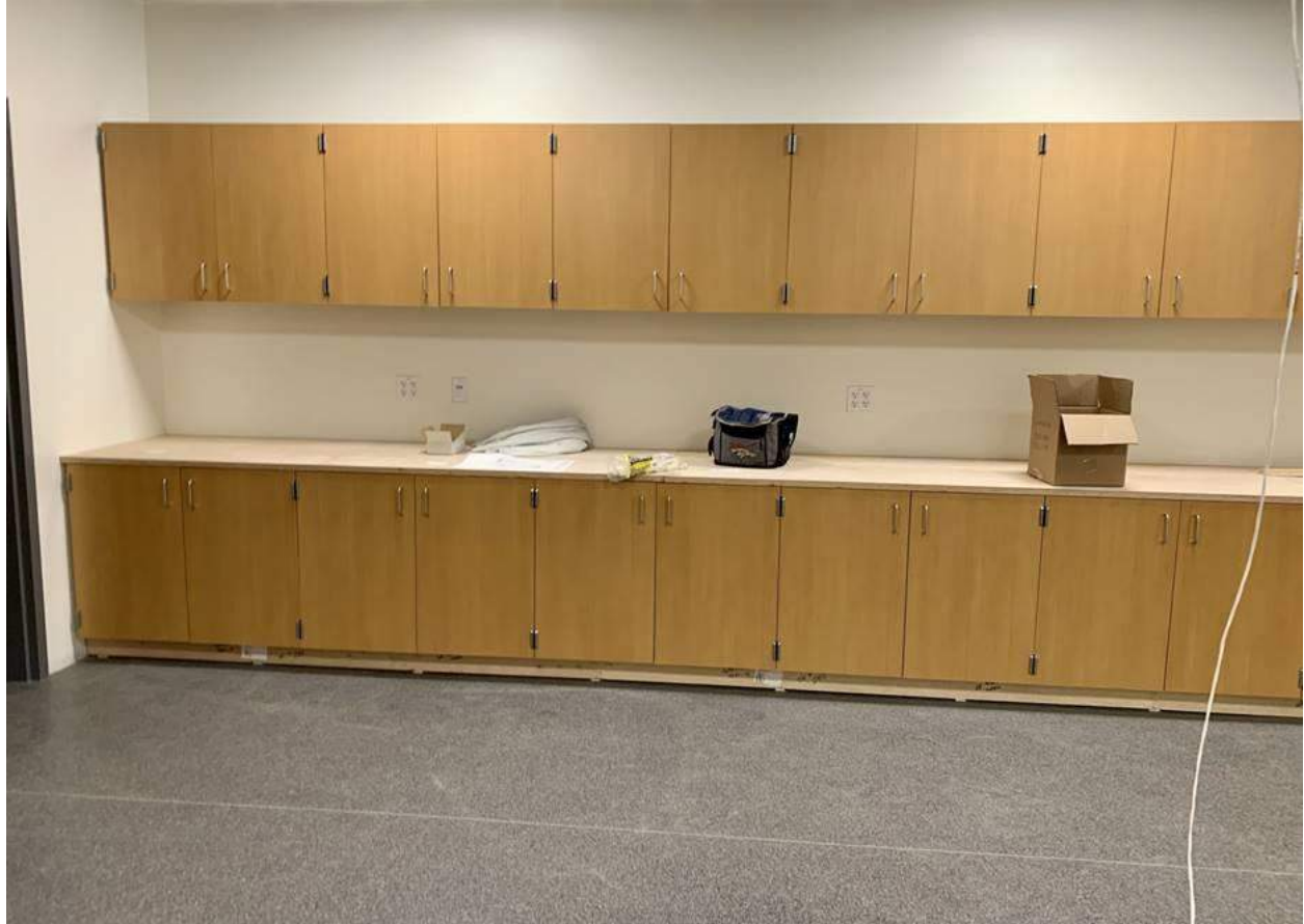
New Admin casework is going in
