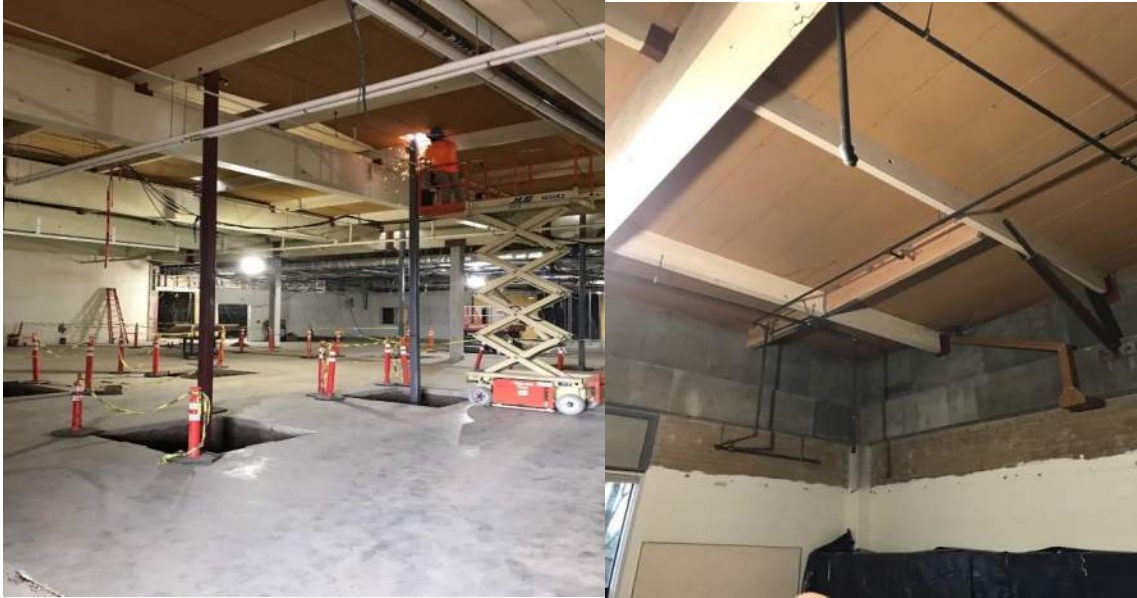
CVHS – Wood shop added columns and Mech room roof improvements
