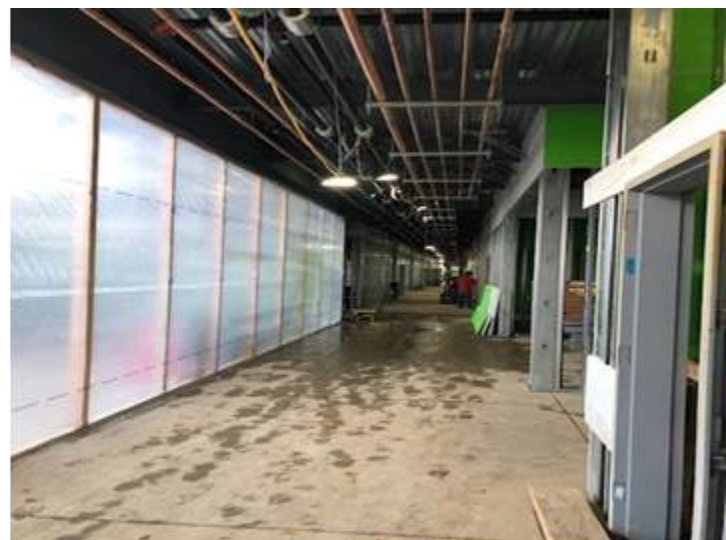
Interior framing and mechanical work underway
