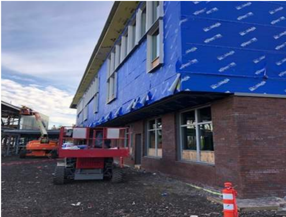
Exterior skin to insure the school is water tight
