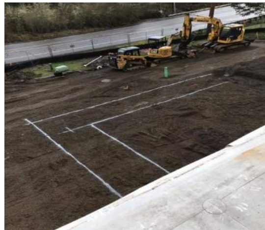
CVHS Building expansion painted on ground for footing excavation
