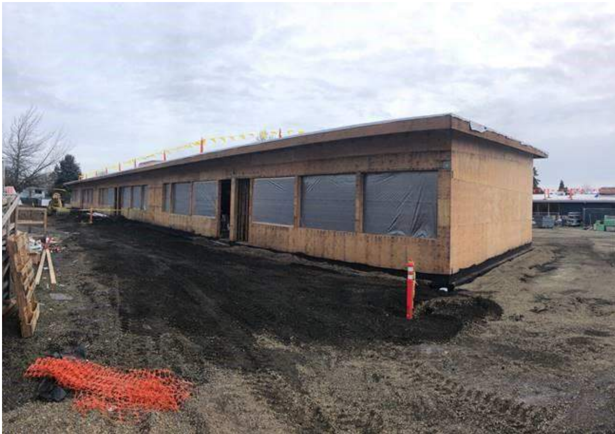
Area C North side framing and temp window protections
