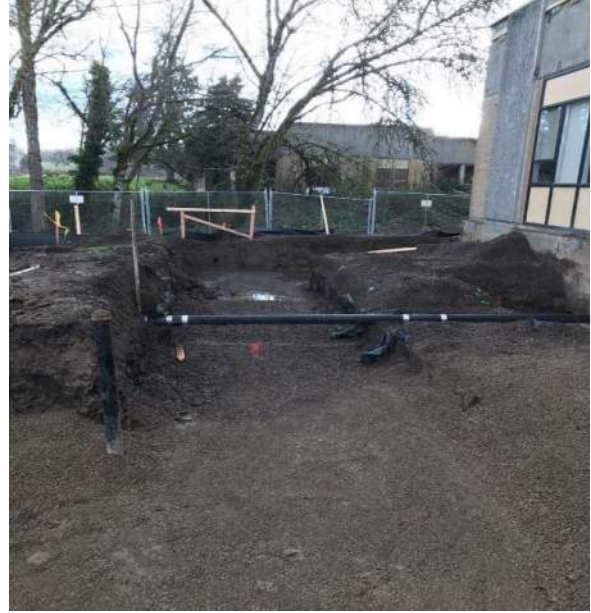
CVHS Outdoor work area – utilities connected and starting footings
