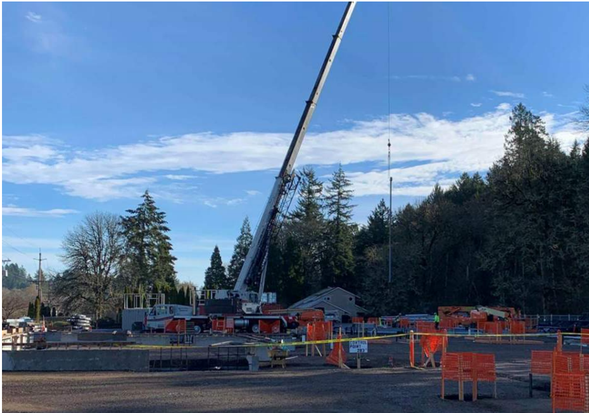
First steel column being set
