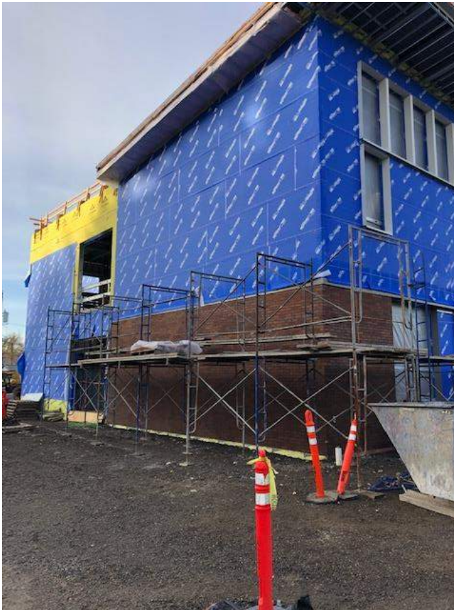
Exterior brick going up
