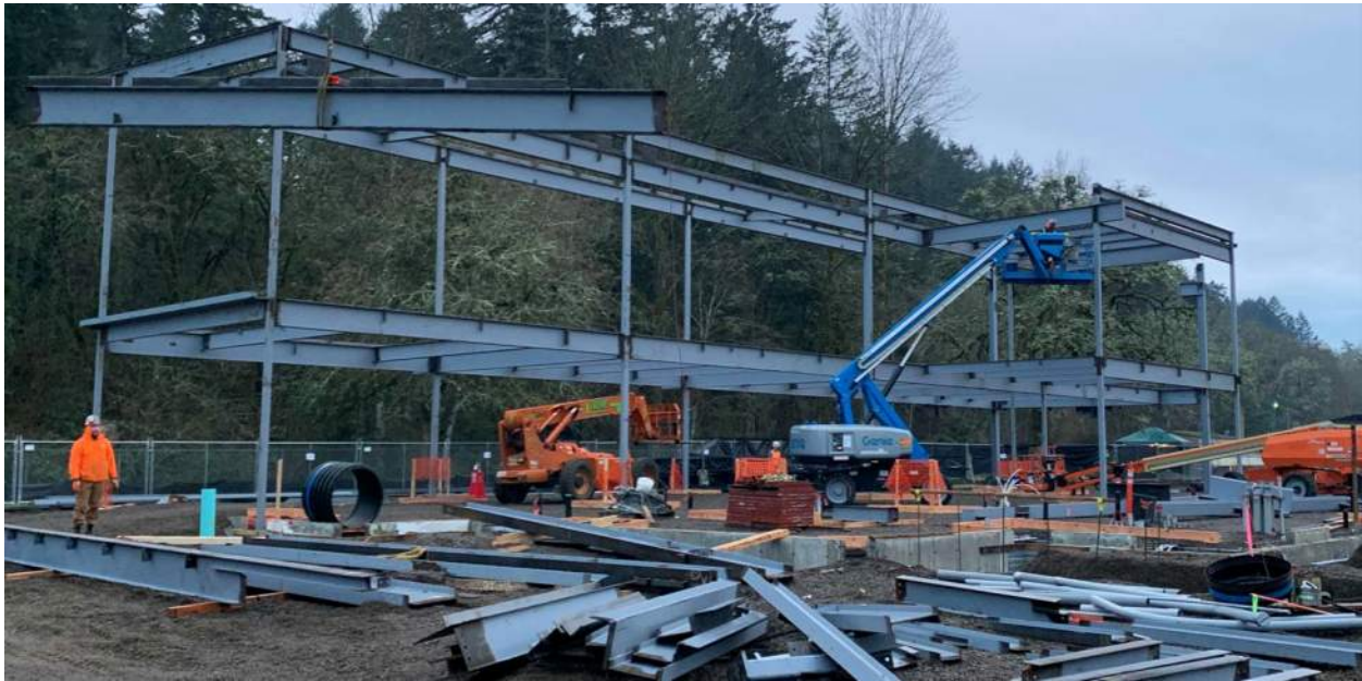
Ongoing structural steel erection
