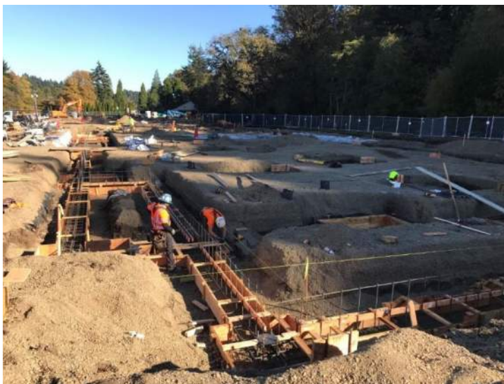
A view of the formwork and rebar
