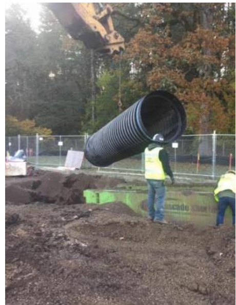
Large storm drainage piping being placed
