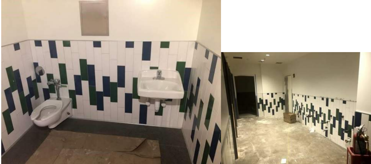
New restrooms – construction progress
