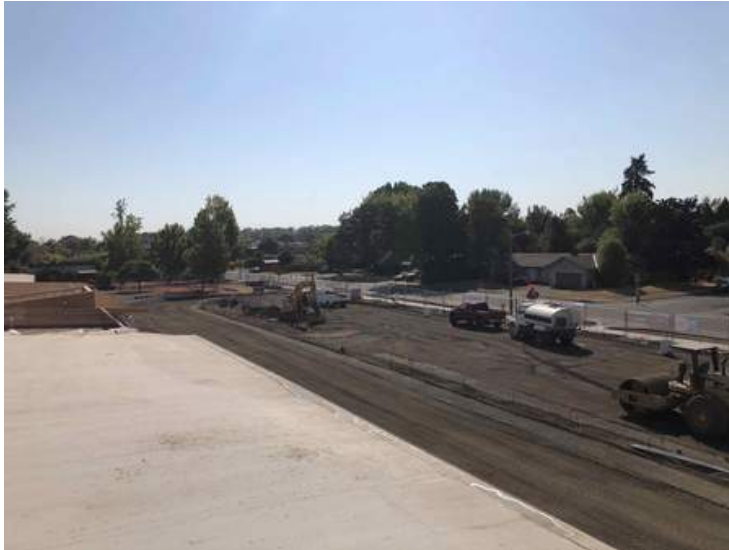
Prep for paving the new parking lot and street work
