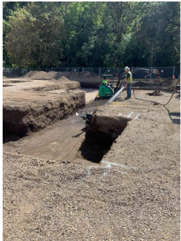
Adding water for better compaction and dust control
