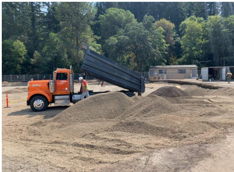
Removing soft soils and replacing with compacted gravel
