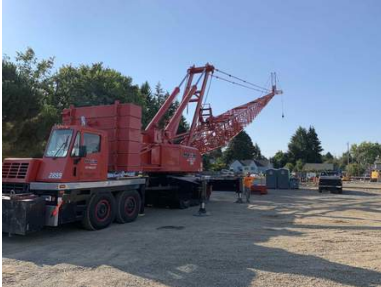
Crane arrives for steel erection
