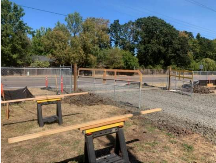
Construction entrance off Walnut
