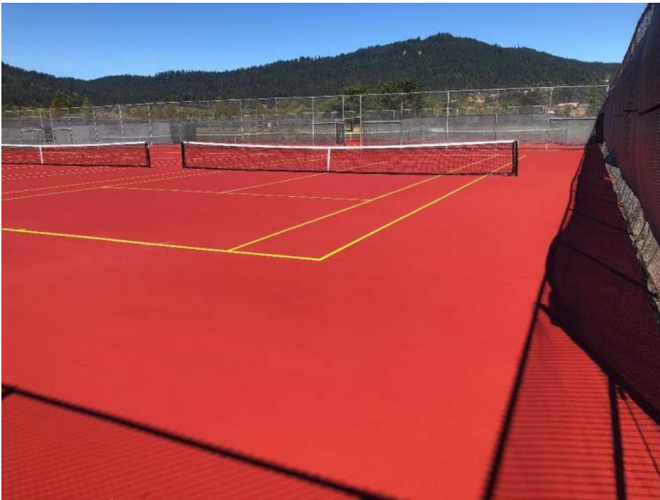
Tennis court resurface work
