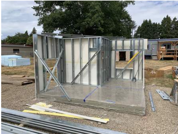
Mockup of polished concrete slab and framing
