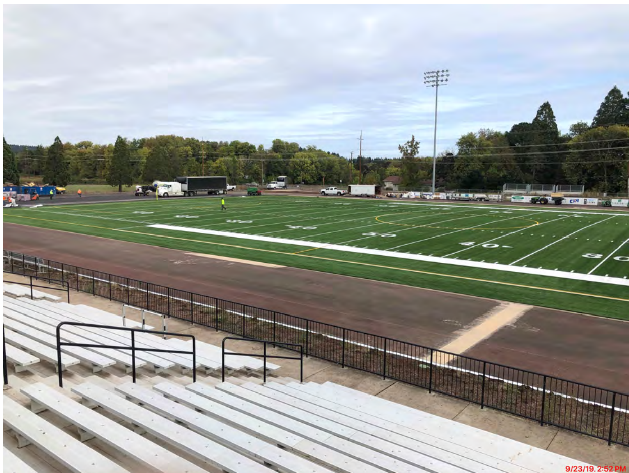
CVHS new turf field is complete
