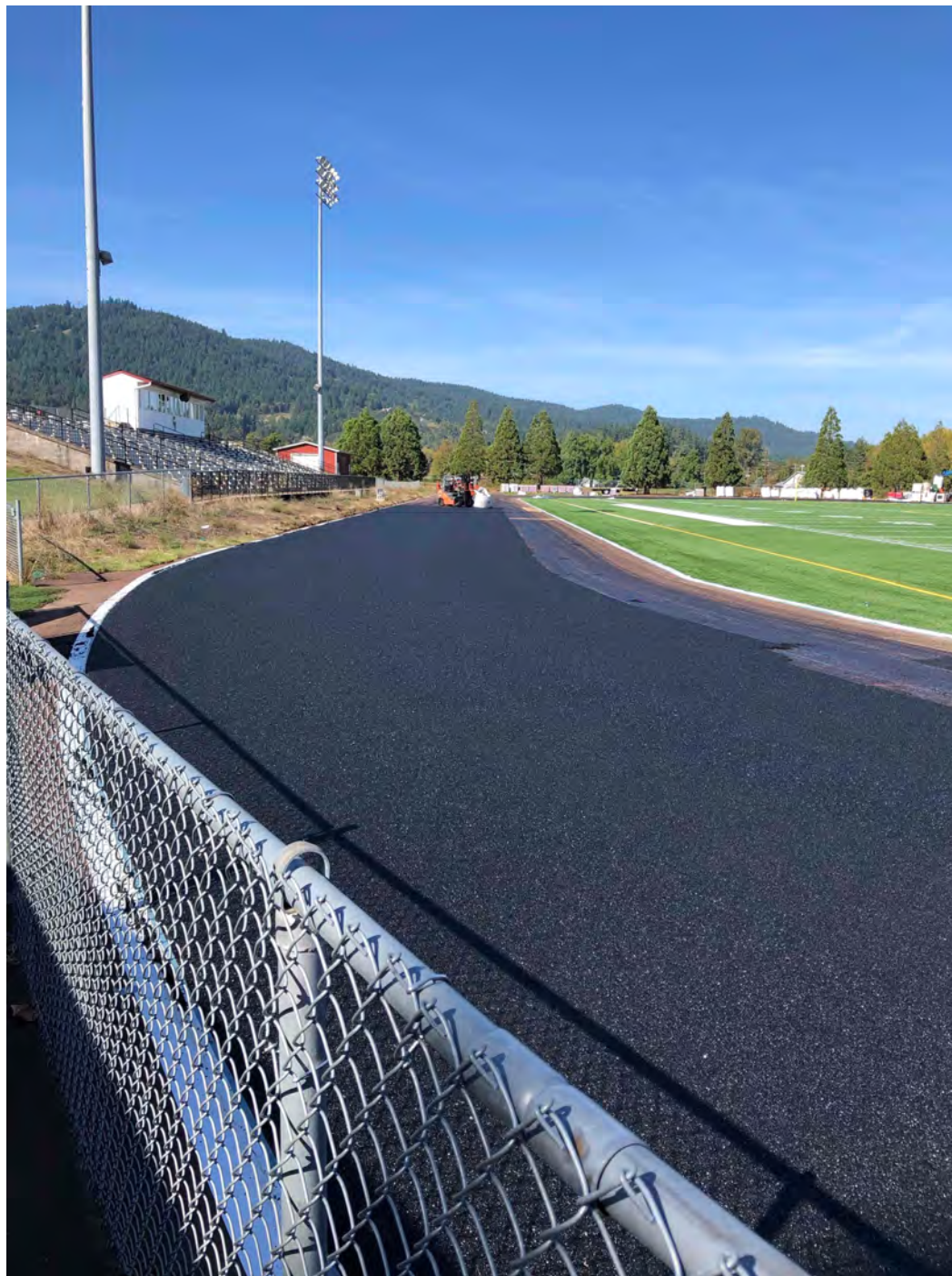
CVHS new track rubber surface going down
