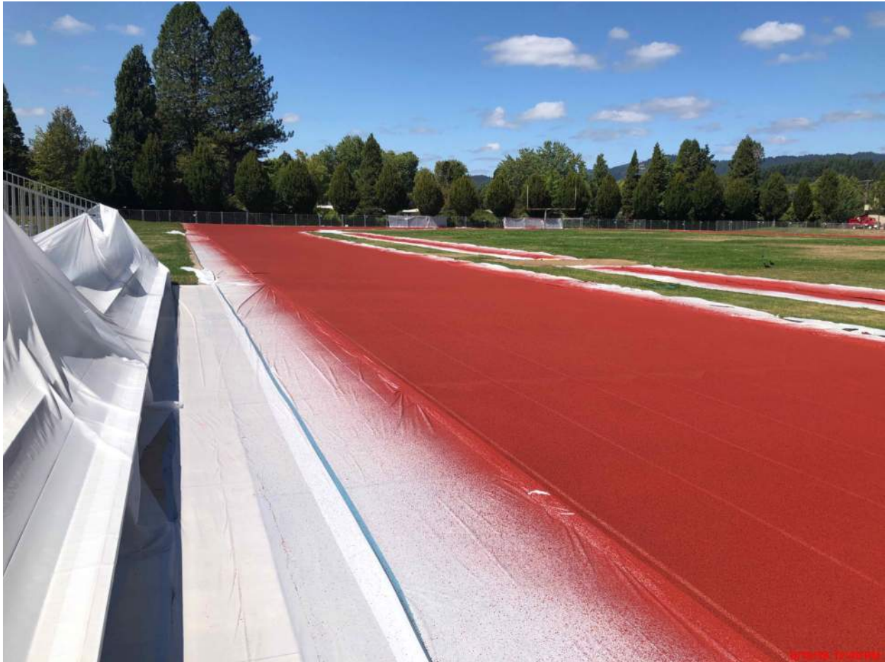
Track surface being applied
