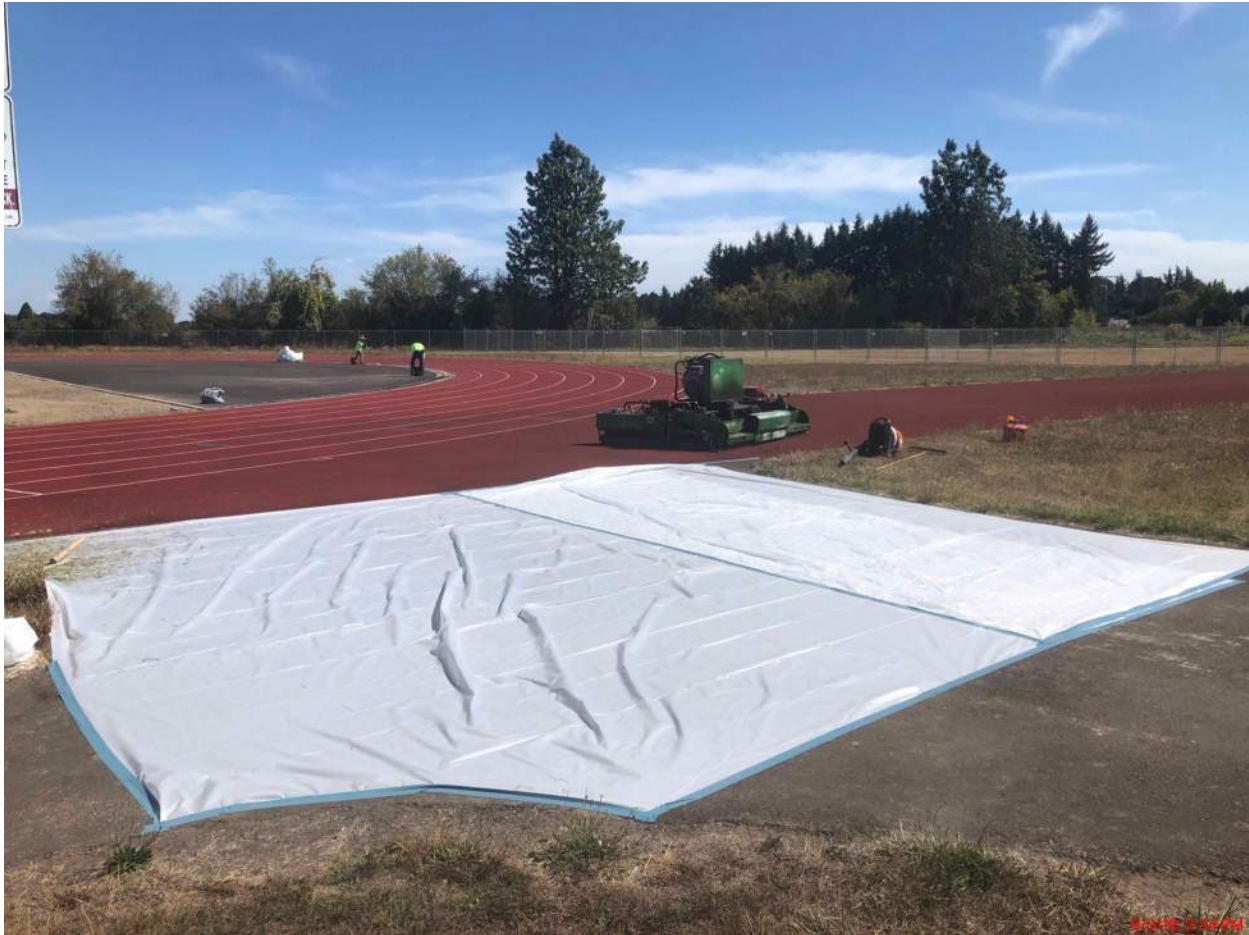
Track Resurfacing begins
