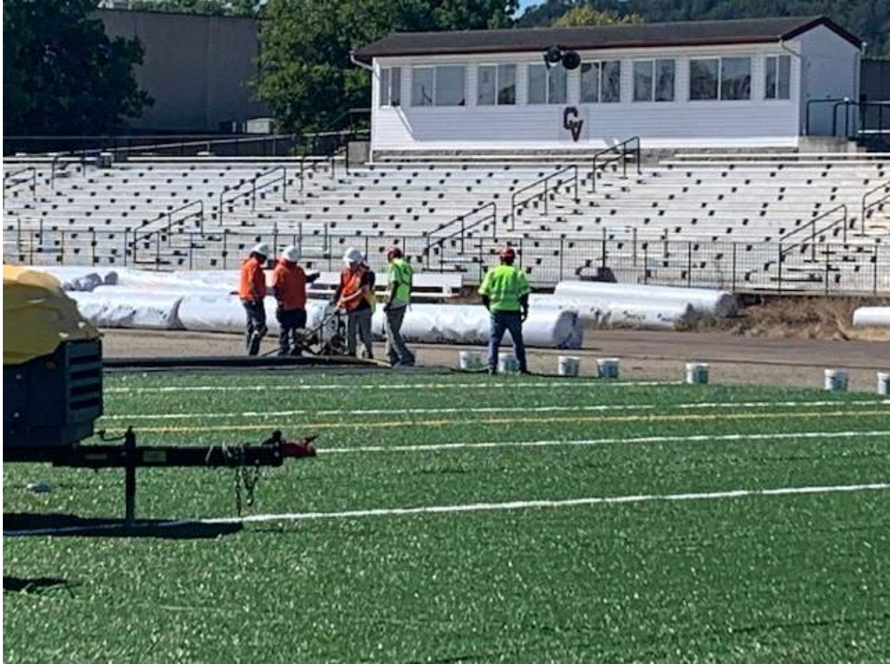
Shaw turf installation begins
