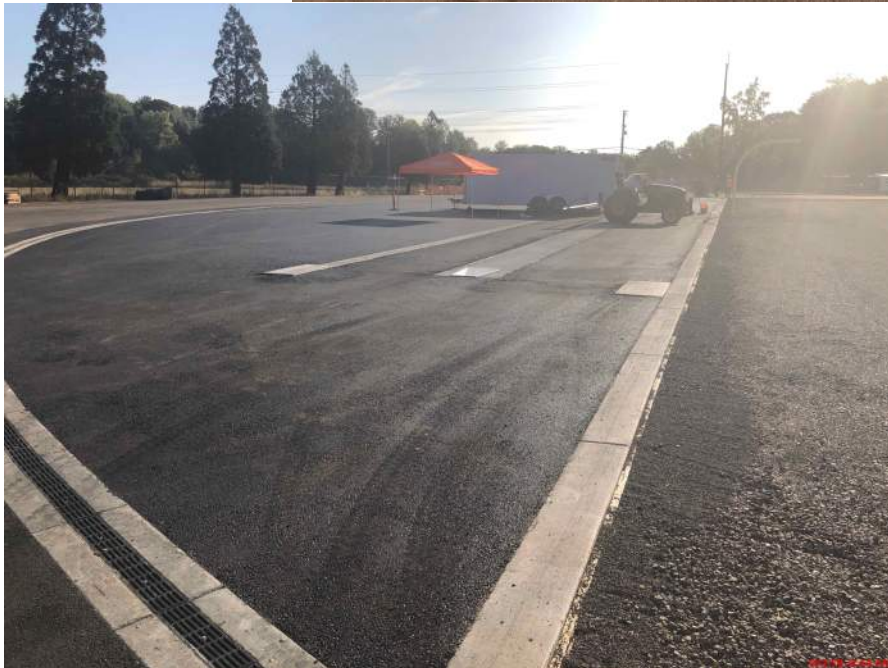
CVHS D Zone paving completed
