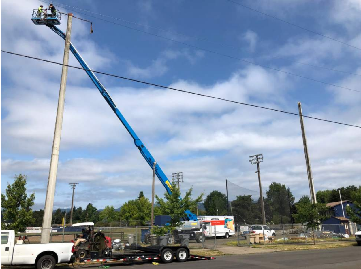
Taylor Field Light replacement
