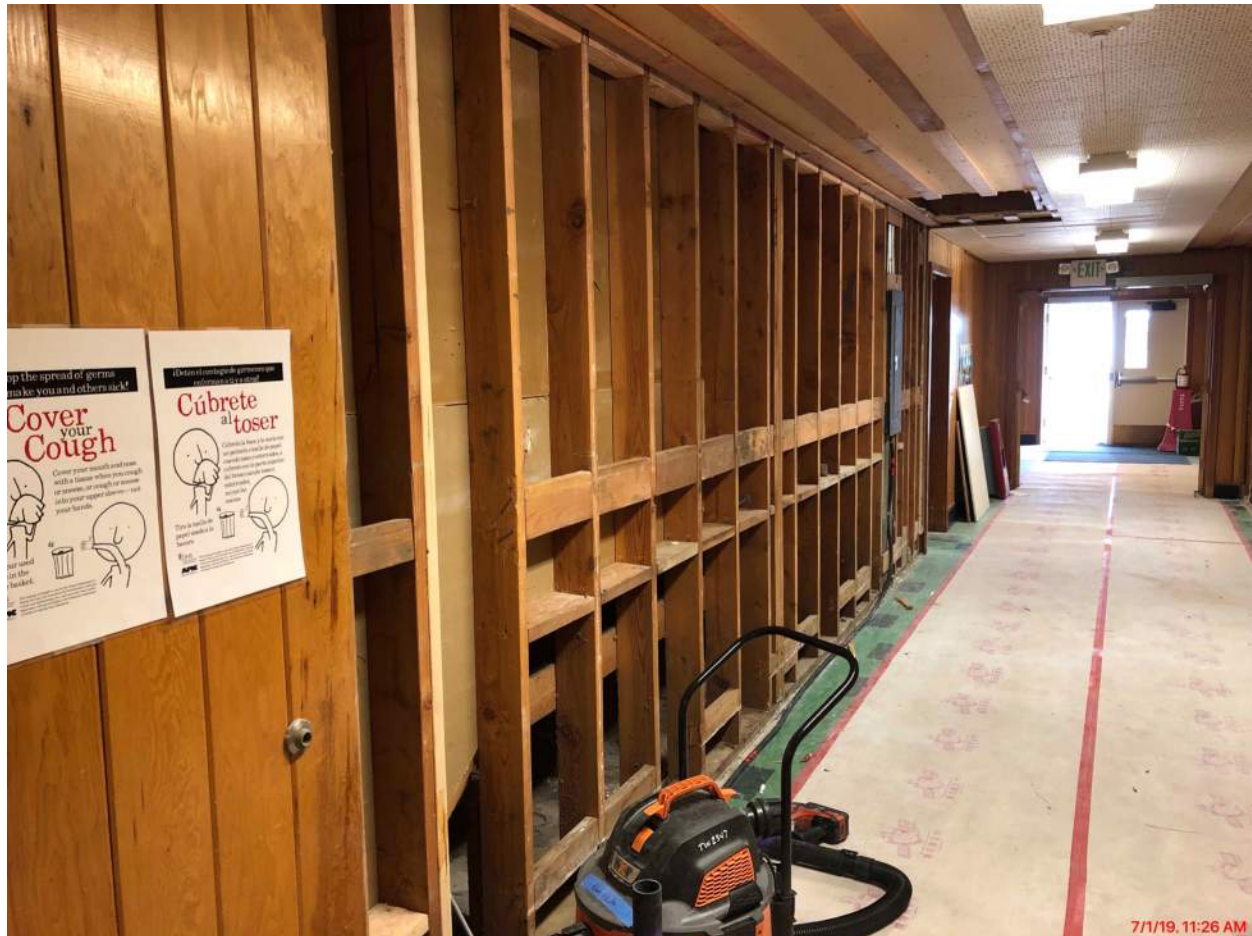
Demolition underway for Jefferson seismic project
