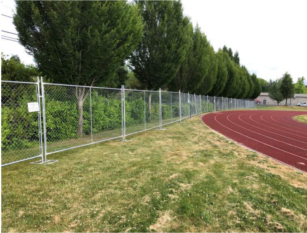
Tree Protection installed
