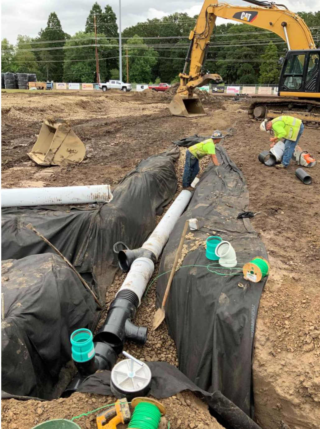
CV Athletics work in progress
