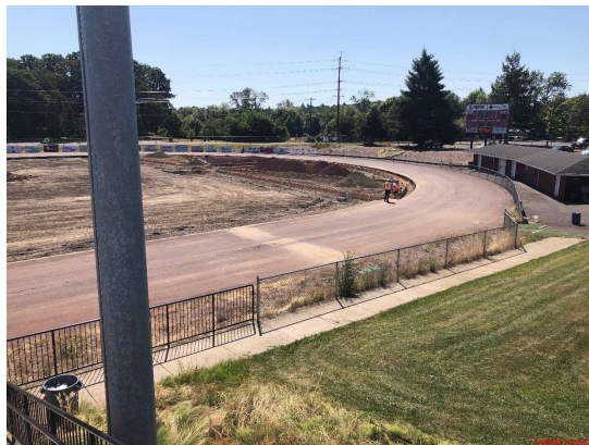
Track and athletic field work underway
