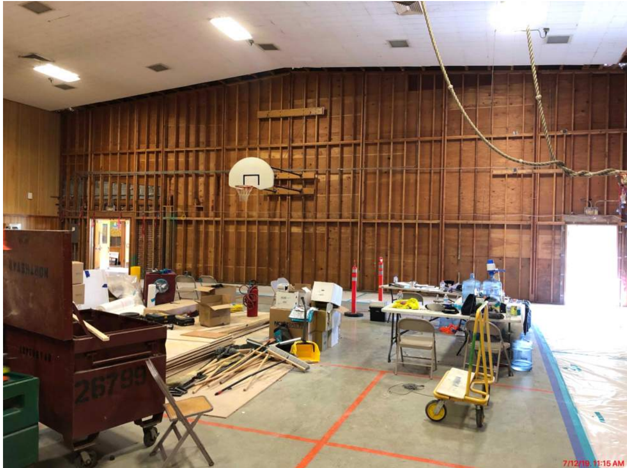
Seismic work at Wilson Gymnasium
