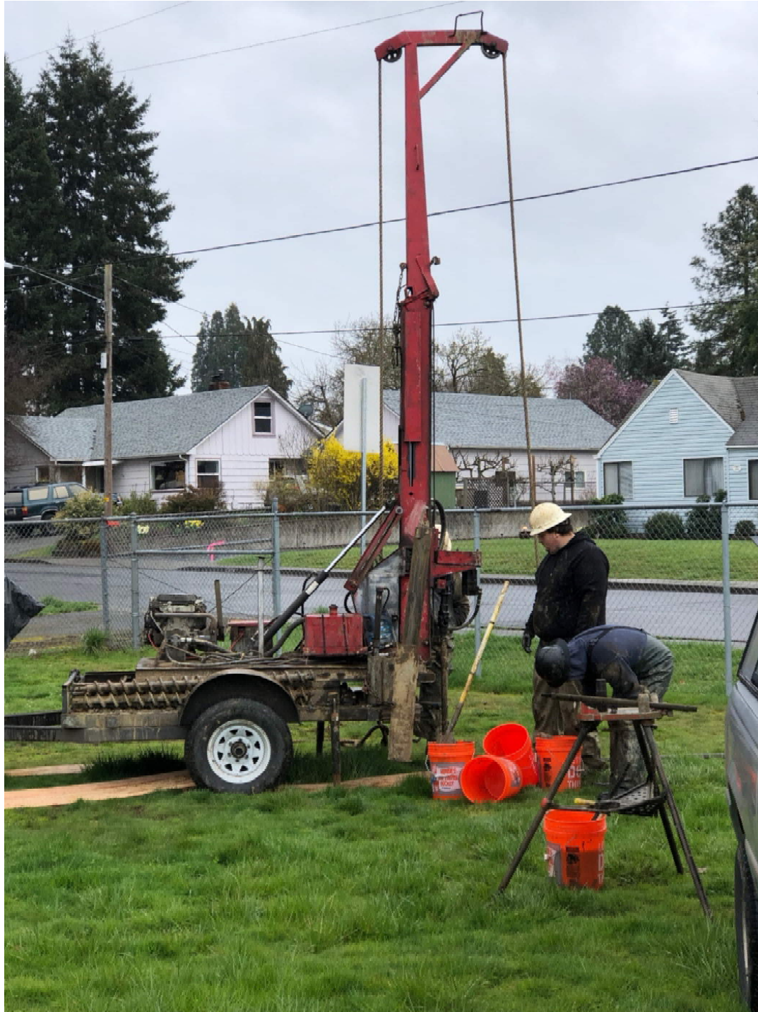
Drilling for the geotechnical survey
