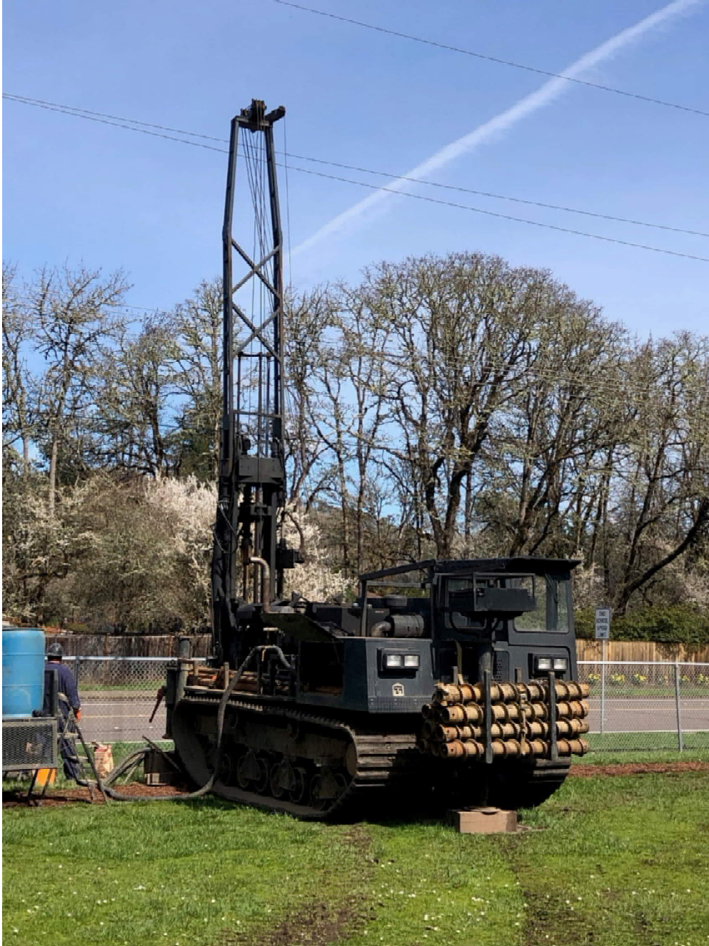
Drilling for geotechnical survey at Hoover Elementary
