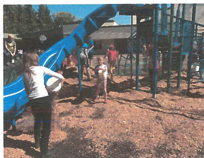
Students helping finish the slide installation.
