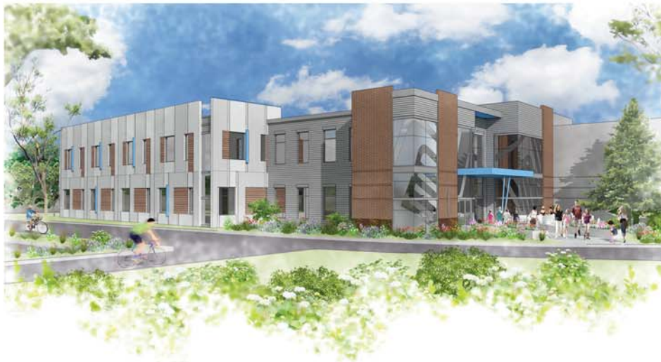
VIEW OF SOUTH-WEST CORNER
