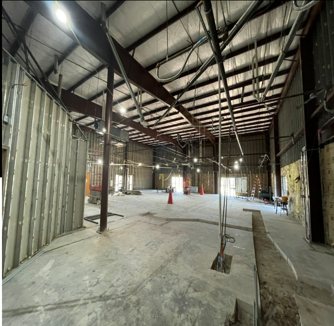
SLAB MEP TRENCH
