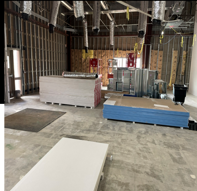
FRAMING - ROUGH-IN - DRYWALL
