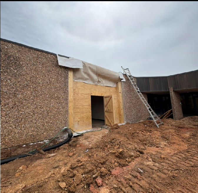
CAFETERIA TEMP PROTECTION
