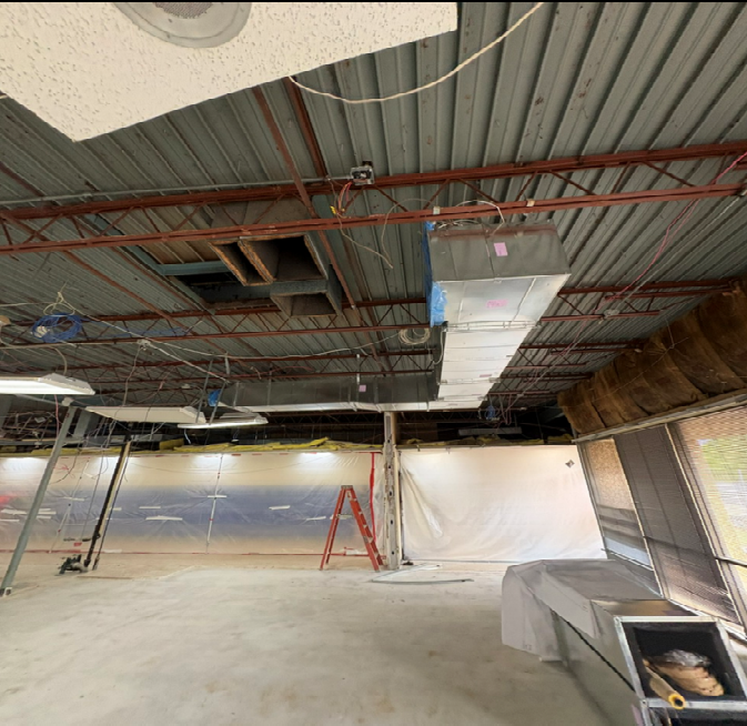
ADMIN CEILING ROUGH-IN
