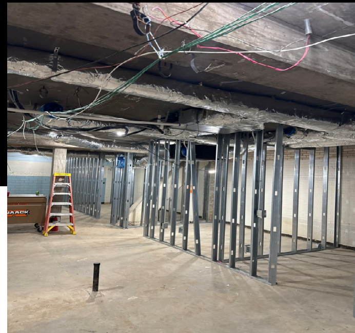
RBE FRAMING - INTERIOR
