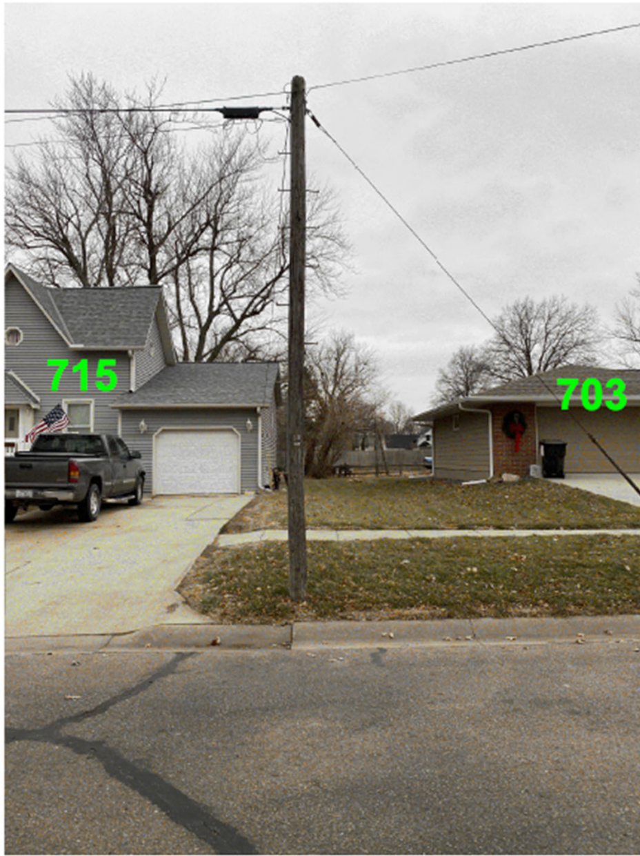
POLE 30NB LOOKING SOUTH
