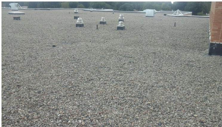
Photo showing additional overview of Area 05 Roof.
