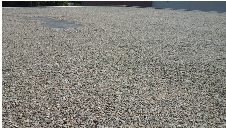
Photo showing overview of Area 24 roof.
