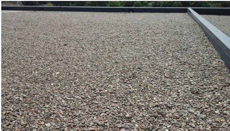
Photo showing additional overview of Area 15 Roof.
