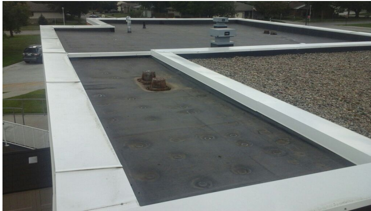
Photo showing overview of Area 06 Roof.
