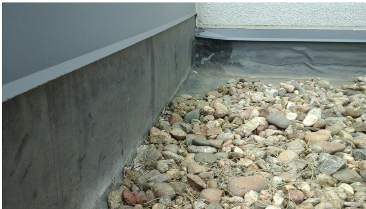
Photo showing condition of the perimeter flashings.
