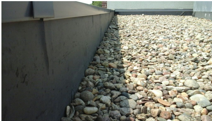
Photo showing condition of the perimeter flashings.
