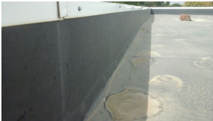
Photo showing condition of the perimeter flashings.
