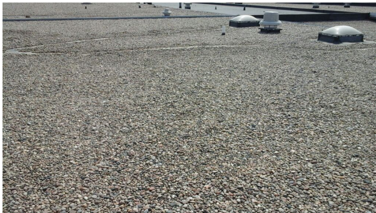
Photo showing additional overview of Area 06.
