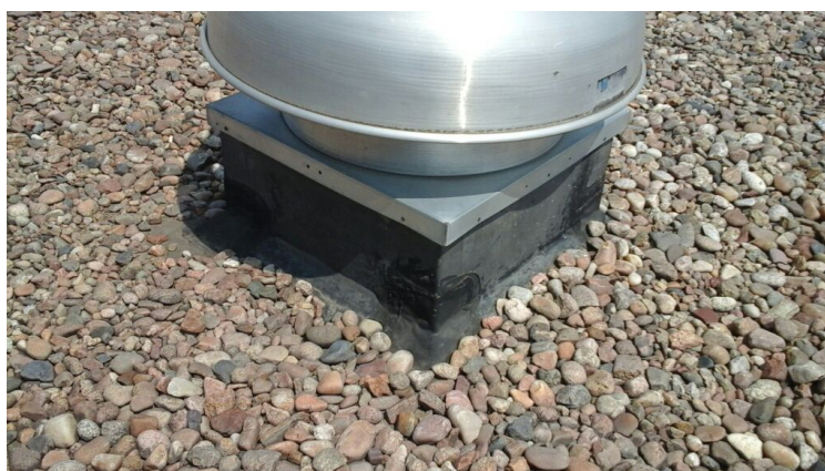
Photo showing condition of projection flashings.
