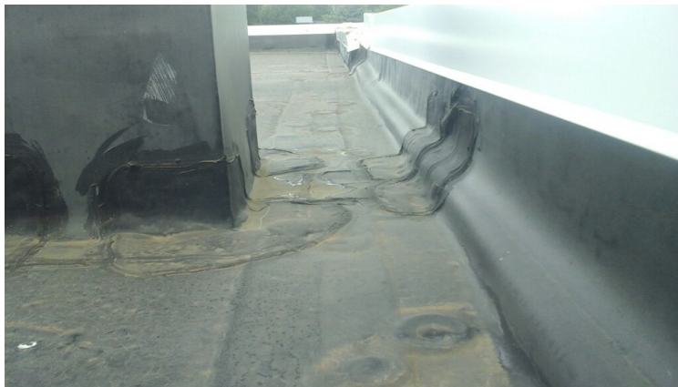
Photo showing condition of the perimeter flashings.
