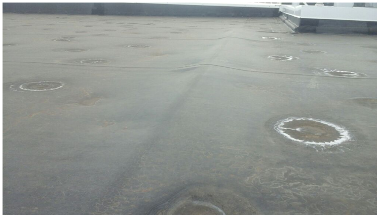
Photo showing coverboard extruding under field membrane due to joints not being staggered on install.
