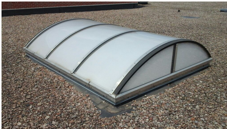
Photo showing condition of the skylight.
