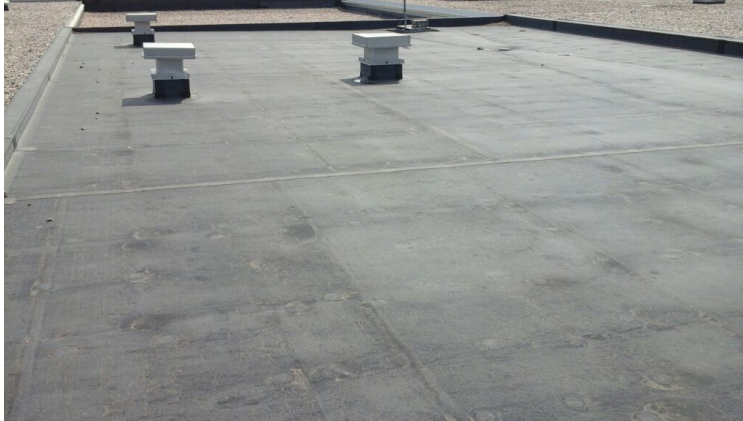
Photo showing overview of Area 07 Roof.
