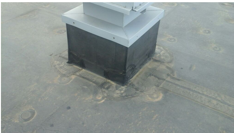
Photo showing condition of projection flashings.
