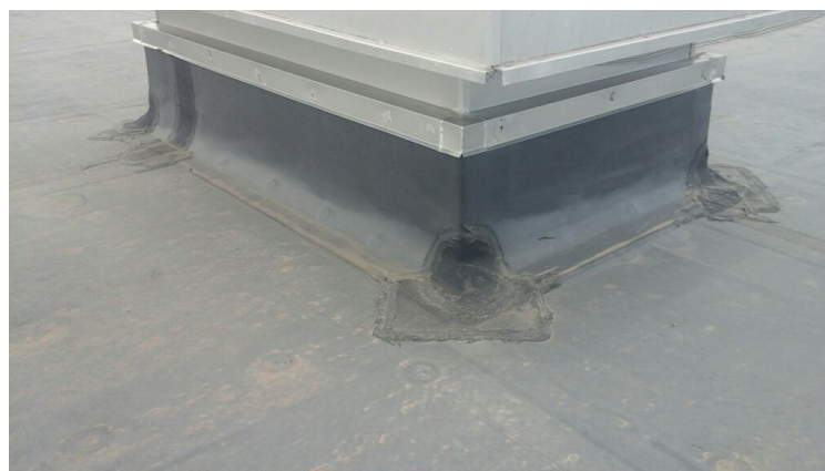
Photo showing condition of projection flashings.
