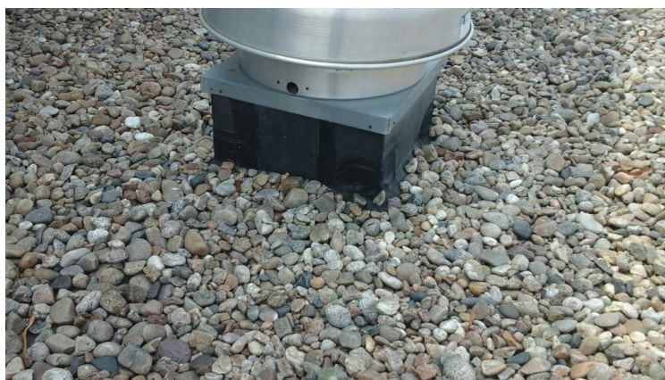
Photo showing condition of projection flashings.
