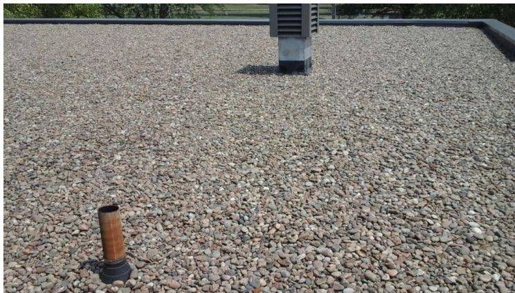
Photo showing additional overview of Area 21 Roof.
