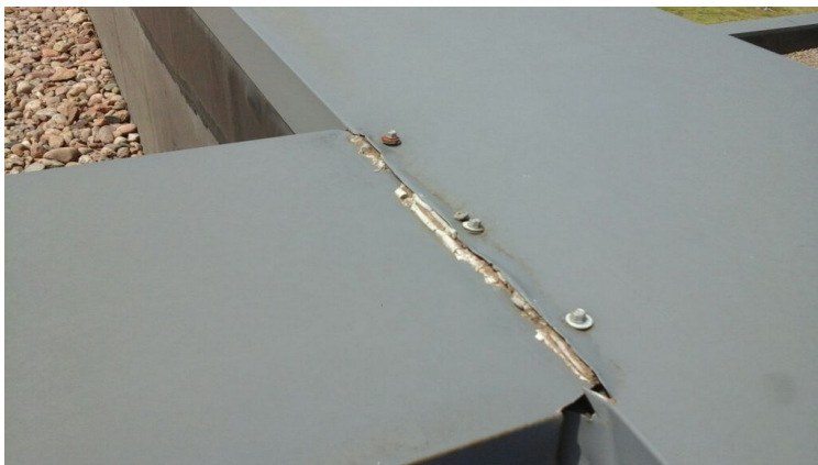
Photo showing caulking beginning to deteriorate on metal.
