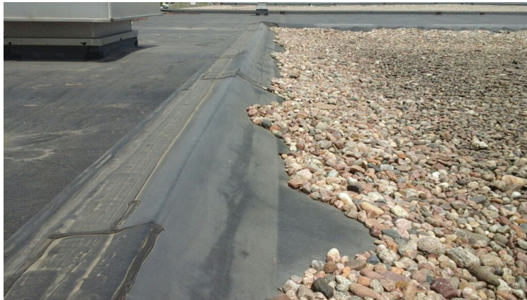
Photo showing condition of expansion joint.
