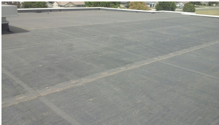
Photo showing additional overview of Area 10 Roof.
