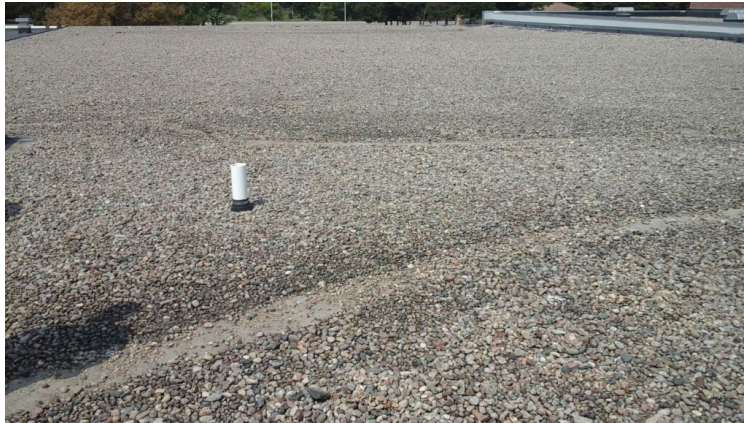
Photo showing overview of Area 06 Roof.
