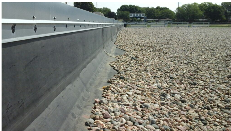
Photo showing condition of the perimeter flashings.
