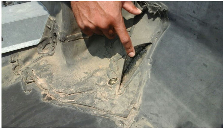
Photo showing additional blowout patch pulling loose.
