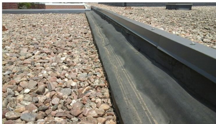
Photo showing condition of the expansion joint.
