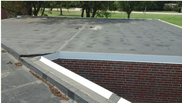
Photo showing additional overview of Area 07 Roof.
