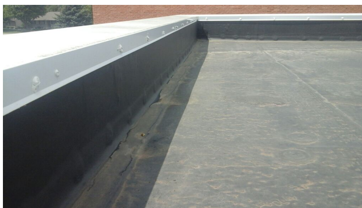
Photo showing condition of the perimeter flashings.
