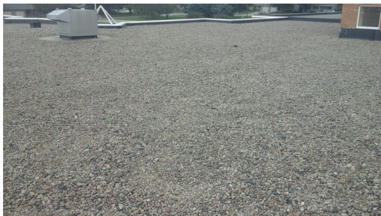
Photo showing additional overview of Area 05 Roof.
