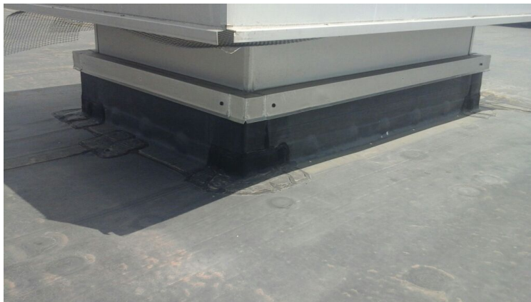
Photo showing condition of projection flashings.
