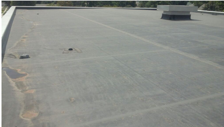
Photo showing overview of Area 10 Roof.
