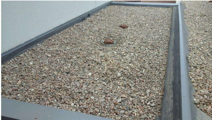
Photo showing overview of Area 12 Roof.
