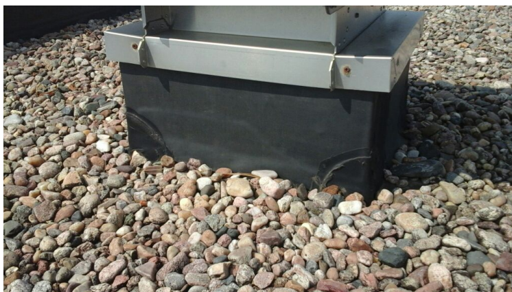
Photo showing condition of projection flashings.
