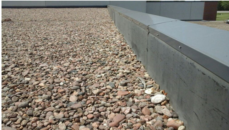
Photo showing condition of the perimeter flashings.
