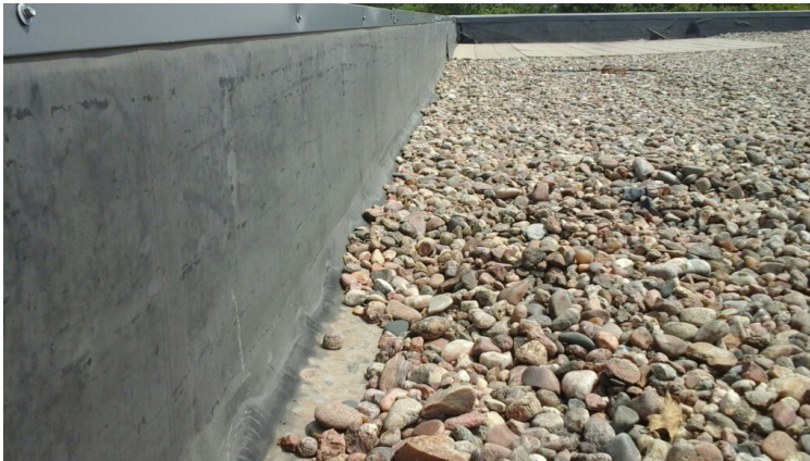
Photo showing condition of the perimeter flashings.
