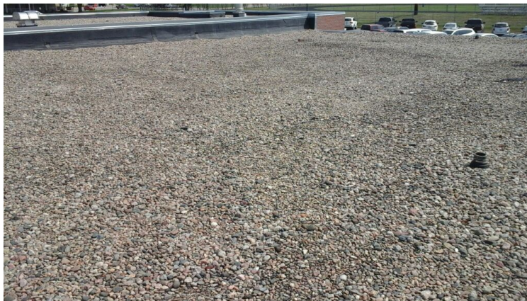
Photo showing additional overview of Area 05 Roof.
