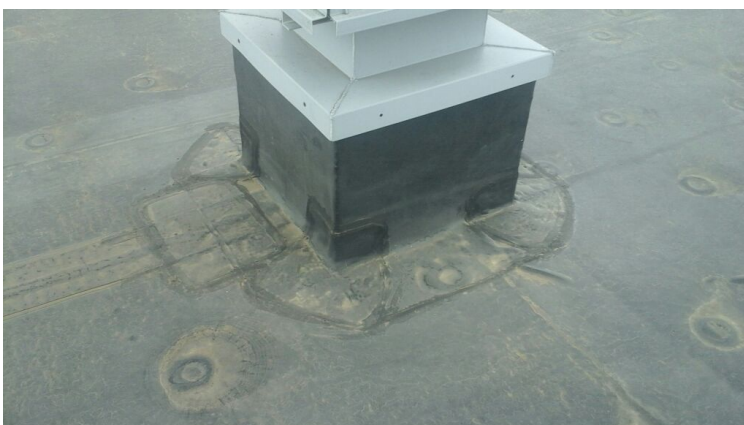
Photo showing condition of projection flashings.
