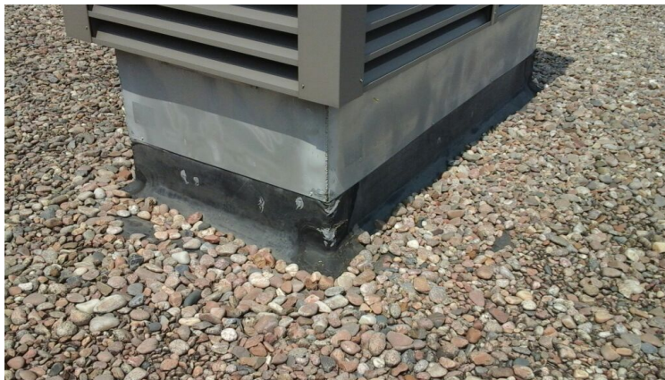
Photo showing condition of projection flashings.
