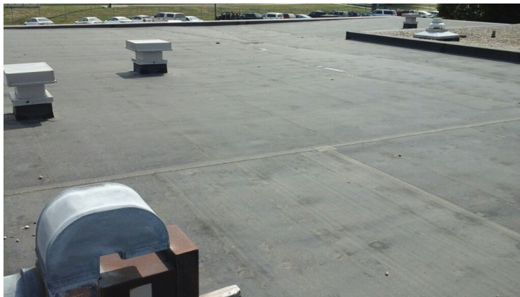
Photo showing additional overview of Area 09 Roof.
