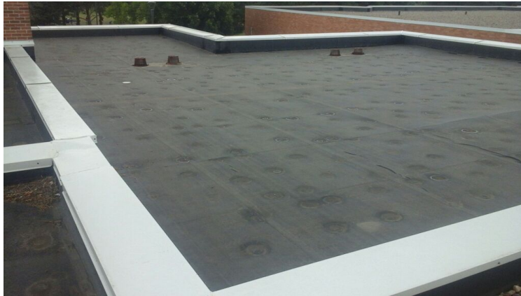
Photo showing overview of Area 04 Roof.
