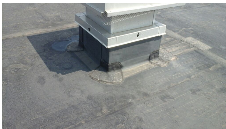
Photo showing condition of projection flashings.
