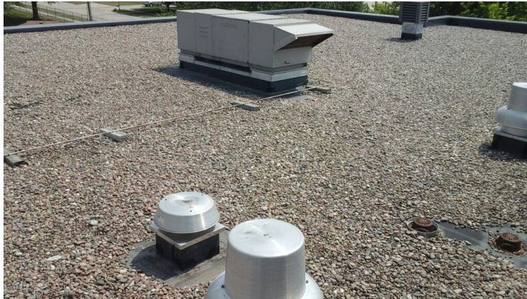
Photo showing overview of Area 21 Roof.
