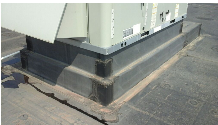
Photo showing condition of projection flashings.
