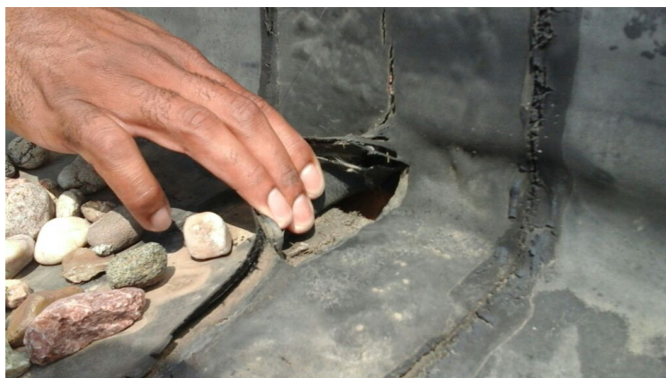
Photo showing a hole in the perimeter flashing. The decking is exposed and this is almost certainly a leak.
