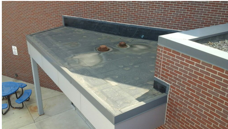
Photo showing overview of small Fully-adhered EPDM area adjacent to Area 11 Roof.
