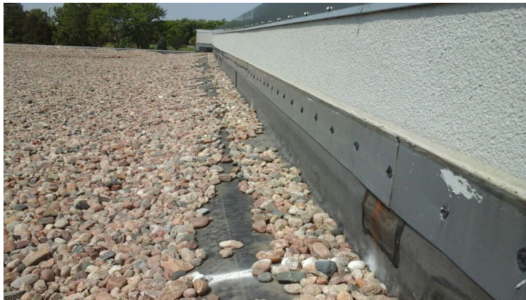
Photo showing condition of the perimeter flashings.
