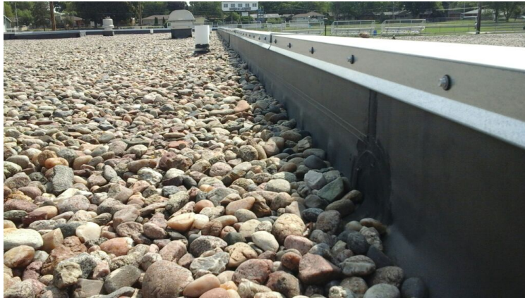
Photo showing condition of the perimeter flashings.
