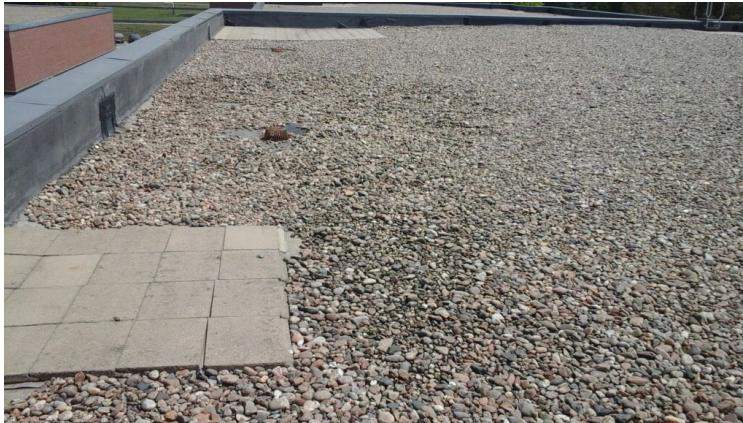
Photo showing overview of Area 15 Roof.
