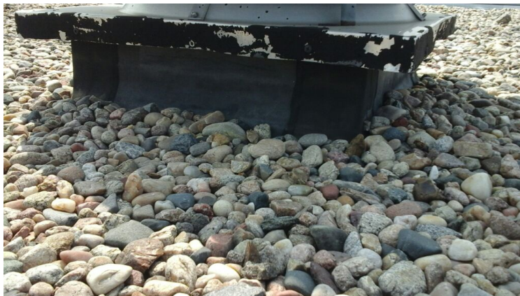
Photo showing condition of projection flashings.
