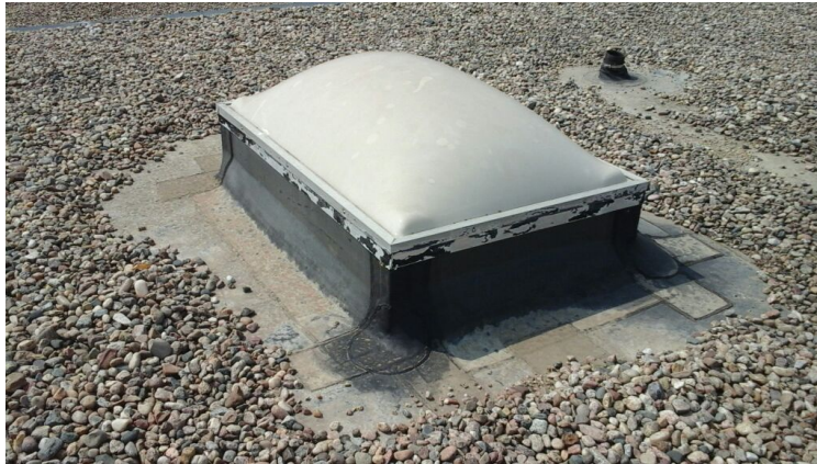
Photo showing condition of the skylights.
