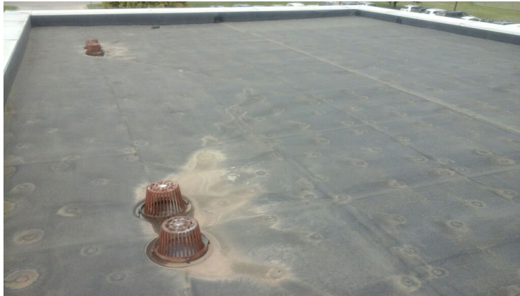
Photo showing overview of Area 01 Roof.
