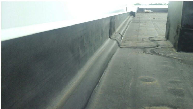
Photo showing condition of the perimeter flashings.
