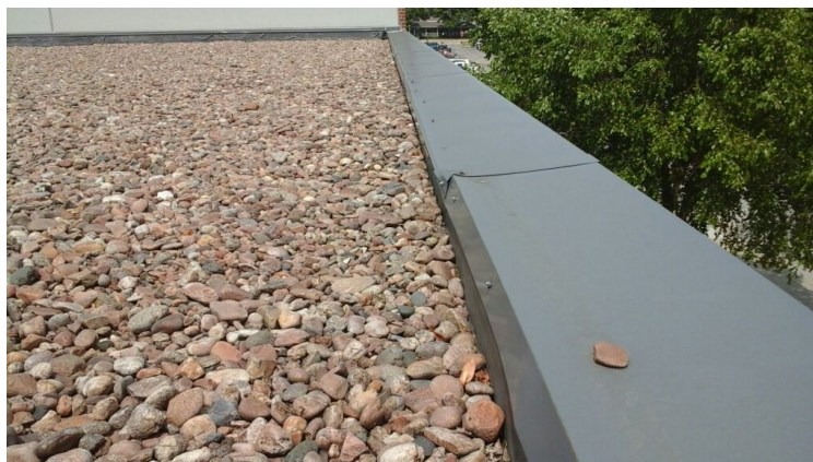
Photo showing mismatched metal sizes.
