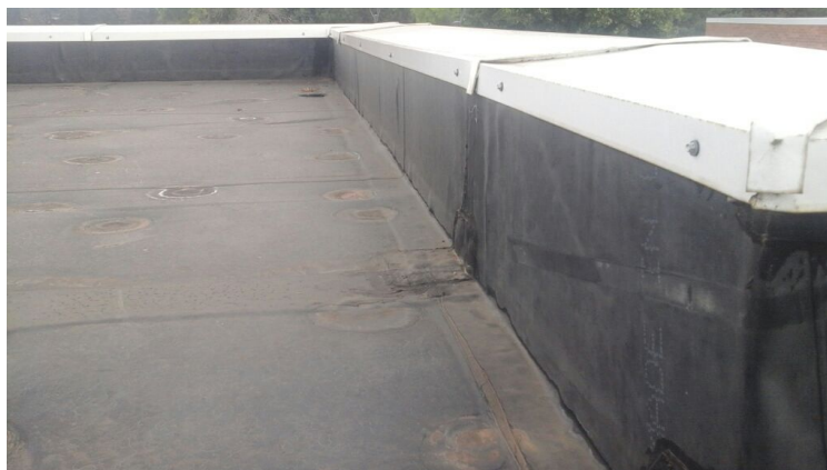
Photo showing condition of the perimeter flashings.
