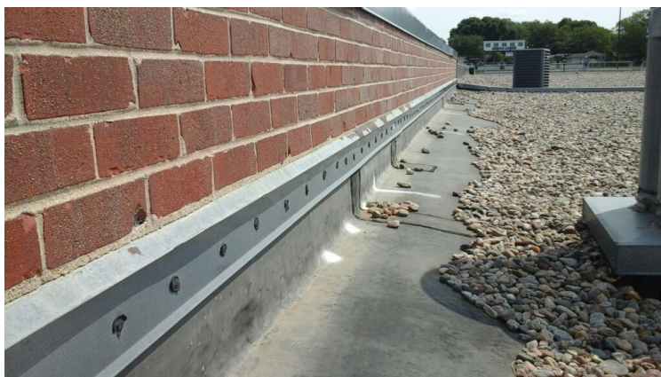
Photo showing condition of the perimeter flashings.
