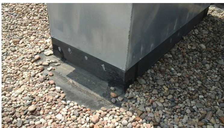
Photo showing condition of projection flashings.
