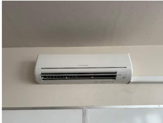
Figure 8 Split-system AC units serve the IT office and server room to provide cooling.
