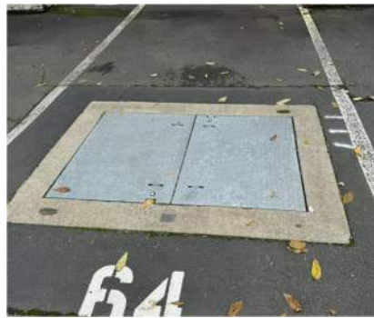
Figure 10 Underground Vault
