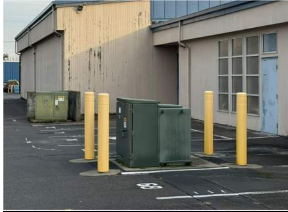
Figure 11 Pad-mounted Transformers
