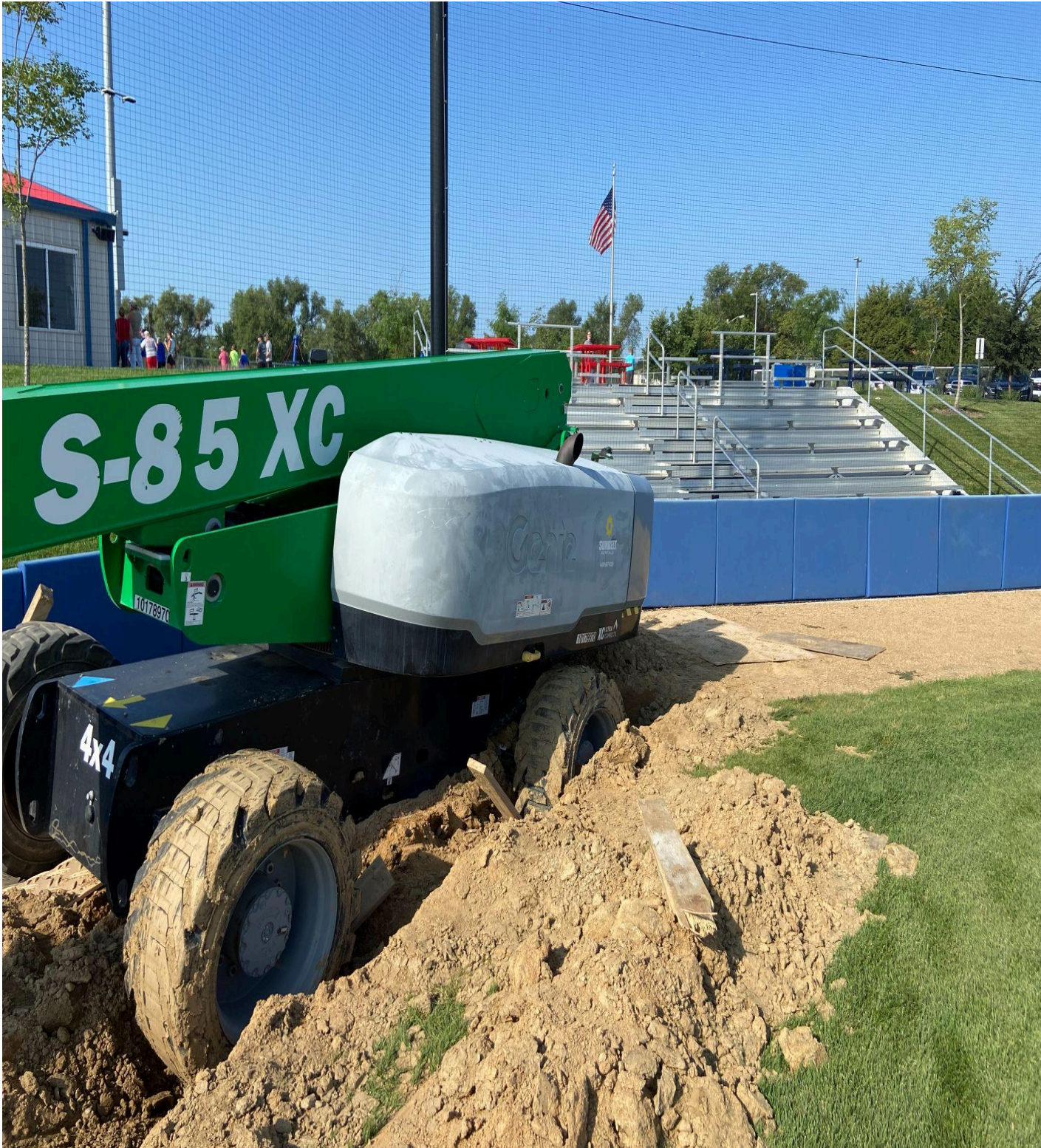
Machine Lift Stuck Behind Home Plate: Facing West
