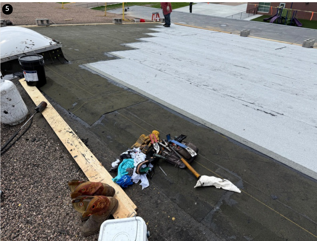
Example of both base and cap sheet being installed. Proper adhesion rates and bleed-out along all lap seams.
