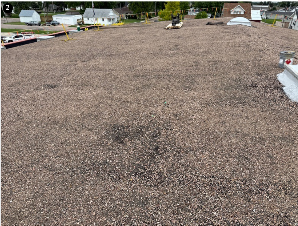
Field overview of roof section during gravel removal.
