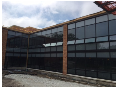
Sprague – Exterior at North
