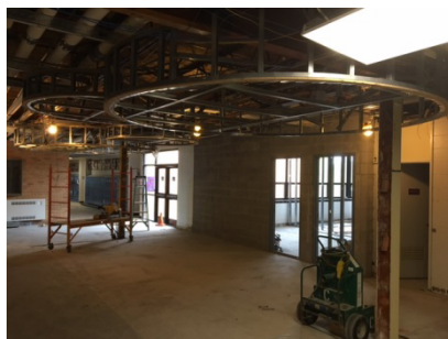
Sprague – Interior/Renovation Space
