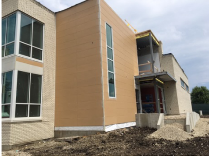
Half Day – Exterior, South Ramp
