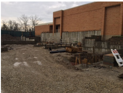
Sprague – East Retaining Wall
