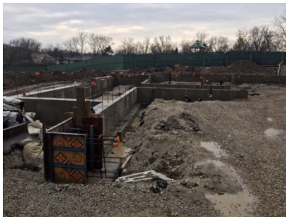
Sprague – West Foundation Walls
