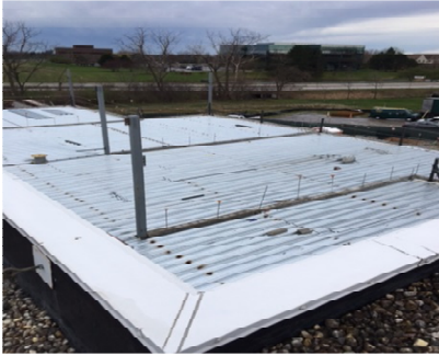
Half Day – Steel Decking
