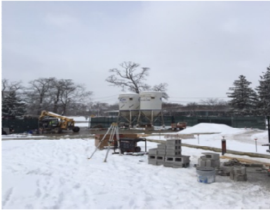
Half Day – Masonry Set-up
