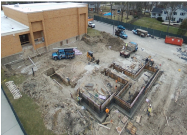
Sprague – Foundations at West
