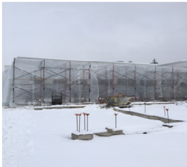
Half Day – Masonry Set-up
