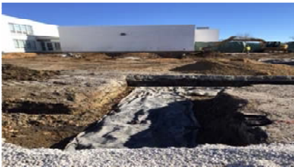
Half Day – Excavation
