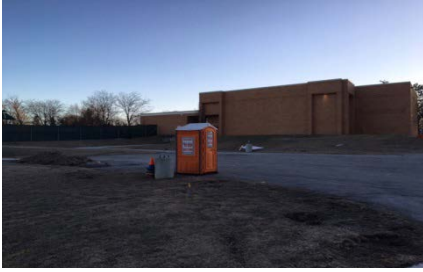
Sprague – Site Clearing
