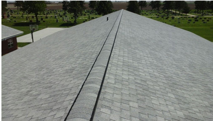
Photo showing overview of Area 01 Roof.
