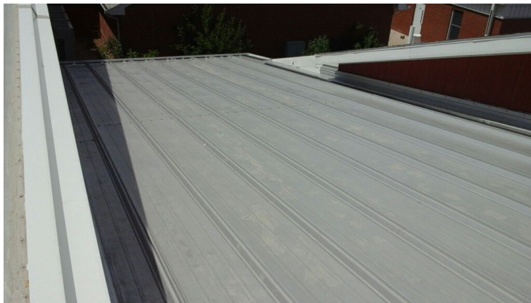
Photo showing additional overview of Area 04 Roof.
