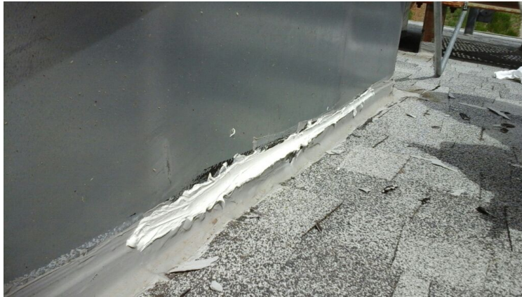
Photo showing temporary repair made to flashing that was exposed.
