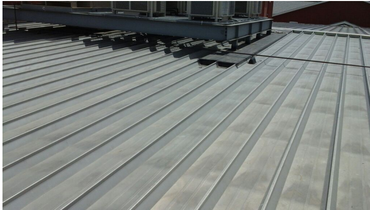
Photo showing overview of Area 12 Roof.
