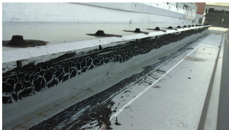
Caulking over tar that pulls right up meaning it is not water tight. This is an area with a leak potentially caused by caulking trapping water where it has failed.
