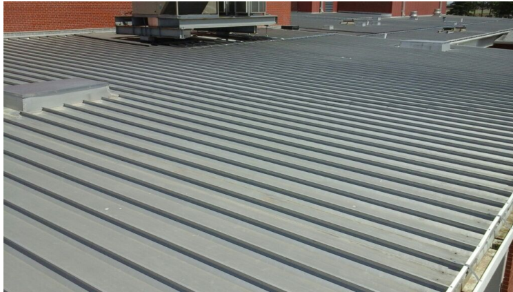
Photo showing overview of Area 08 Roof.
