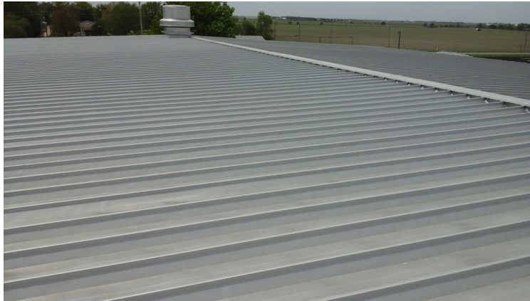
Photo showing overview of Area 16 Roof.
