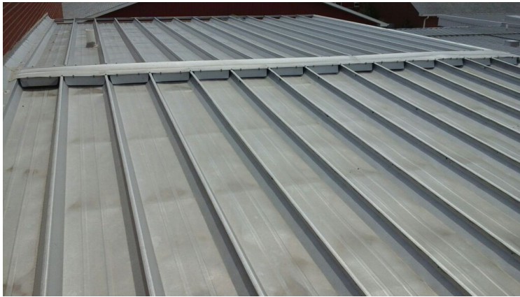
Photo showing overview of Area 14 Roof.
