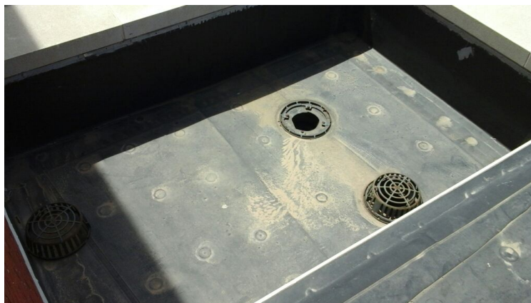
Photo showing additional overview of Area 04 Roof.
