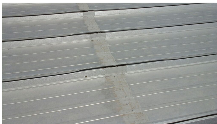
Horizontal seams have been caulked which tends to trap water and pull it through the roof as it deteriorates.
