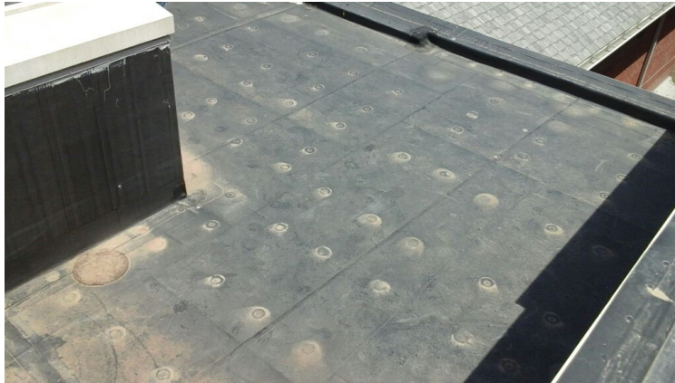
Photo showing additional overview of Area 04 Roof.
