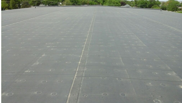
Photo showing overview of Area 02 Roof.
