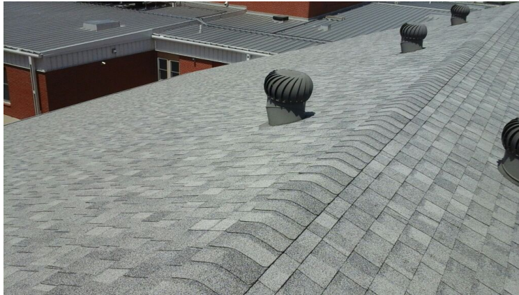
Photo showing overview of Area 03 Roof.
