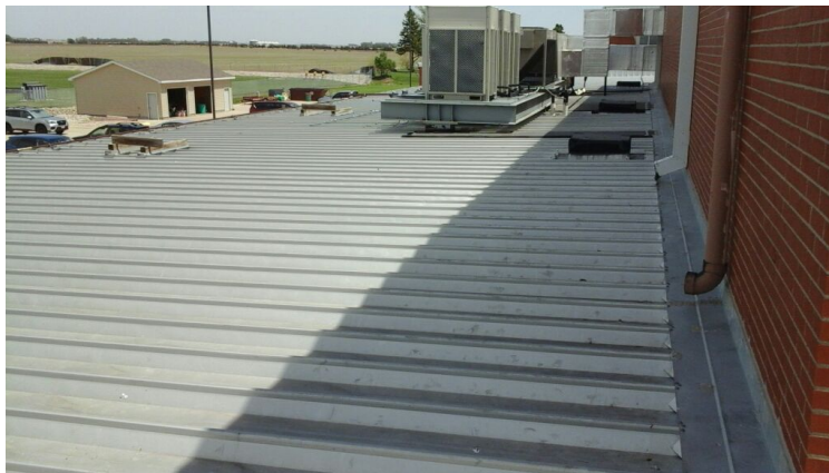
Photo showing additional overview of Area 09 Roof.
