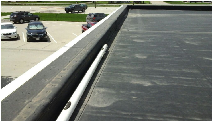
Photo showing condition of the perimeter flashings.
