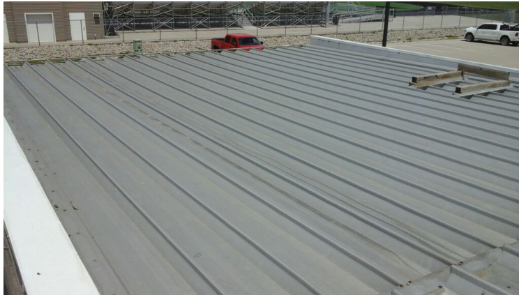
Photo showing overview of Area 11 Roof.
