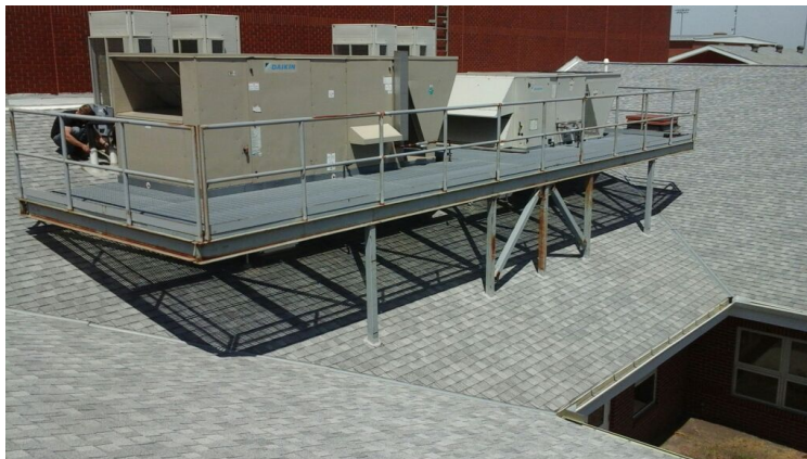
Photo showing additional overview of Area 01 Roof.
