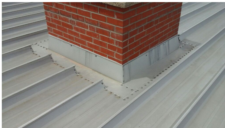
Photo showing condition of projection flashings.
