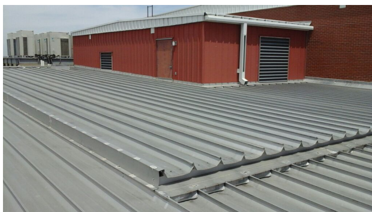
Photo showing additional overview of Area 13 Roof.
