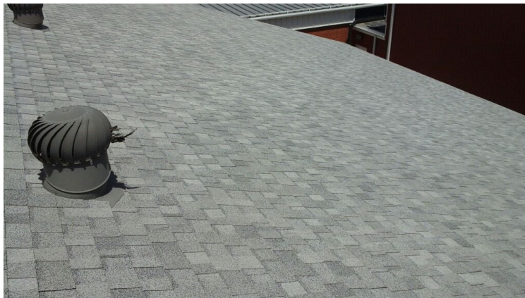
Photo showing additional overview of Area 03 Roof.
