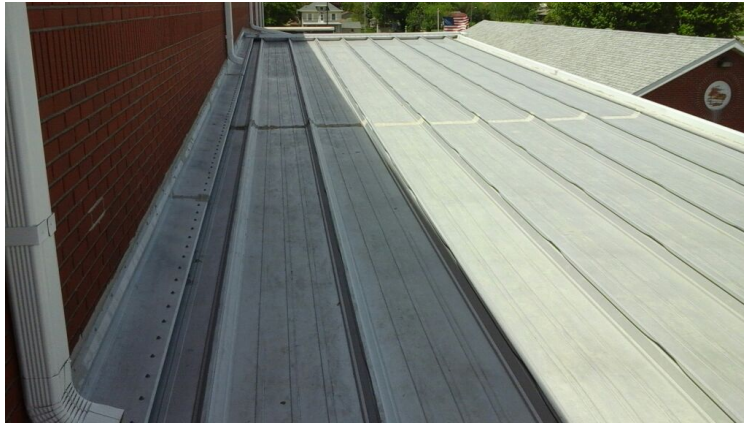
Photo showing overview of Area 04 Roof.
