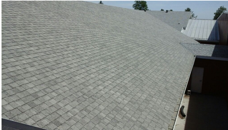
Photo showing overview of Area 07 Roof.
