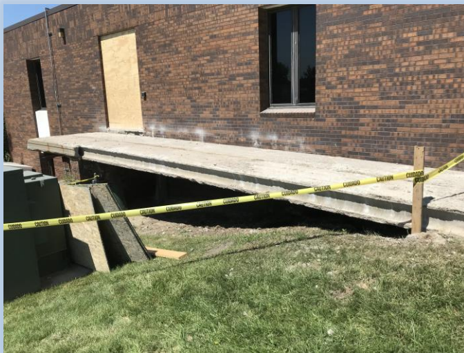
Ramp during construction
