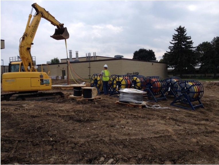
09/02/15 Pulling the new electrical wires for the electrical service.
