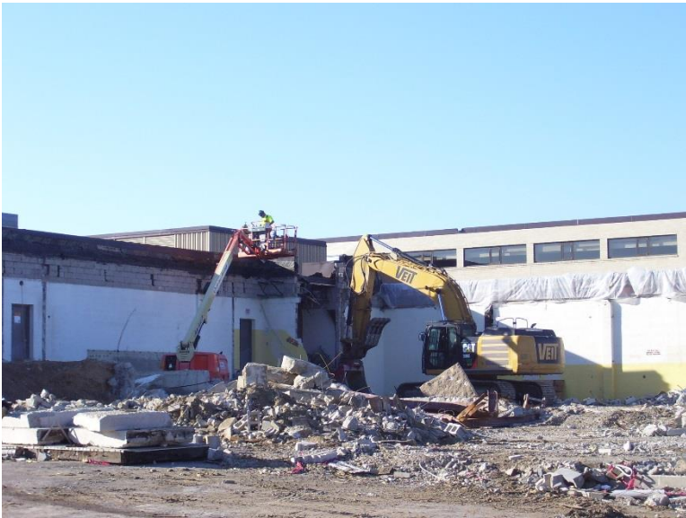
08/10/15 Building demolition of the old Industrial Tech wing.
