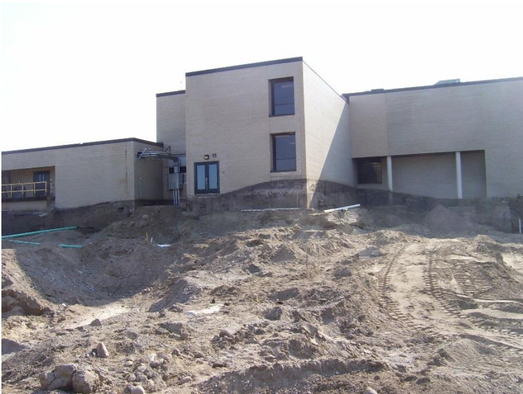
09/15/15 This image shows the amount of excavation at the building pad for the new west addition.
