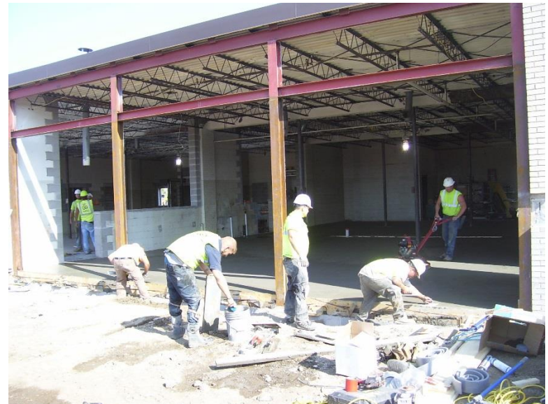
09/05/15 Finishing the new concrete floors in the Annex.
