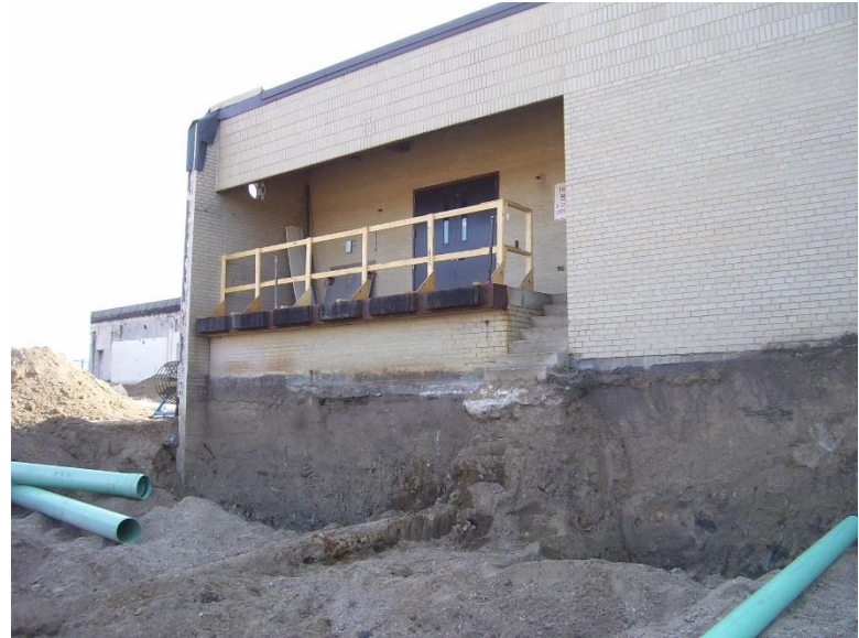
09/15/15 This image shows the depth of subcut at the existing loading dock.
