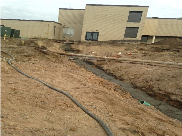
08/27/15 The new underground electrical service being encased in a concrete ductbank.
