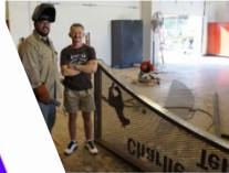
1 Teacher, Vinnie Heller, and Troy Metal Works fabricate the new arch
