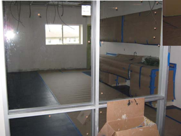
Lobby Area of Falls Career Building
