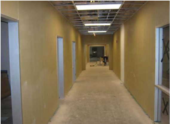
Hallway of East Administration Building
