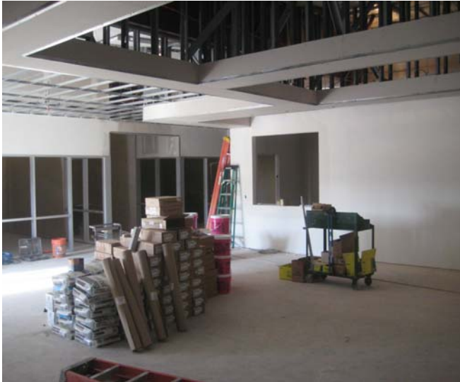
Lobby Area of East Administration Building
