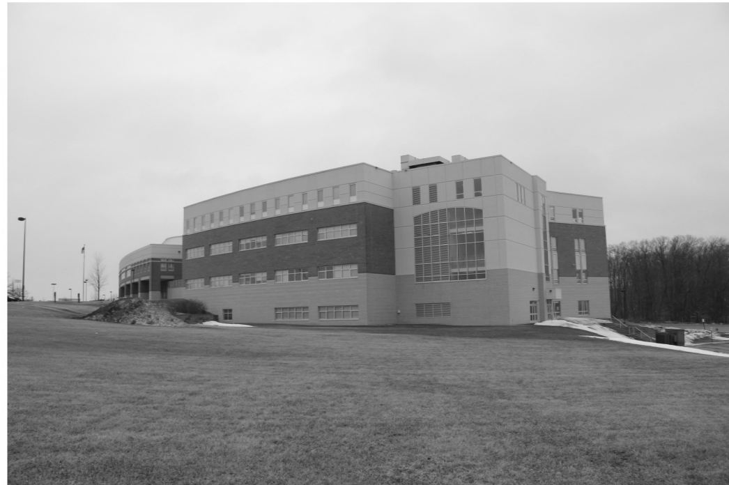
1 EXTERIOR FRONT OF BUILDING (BEFORE)
