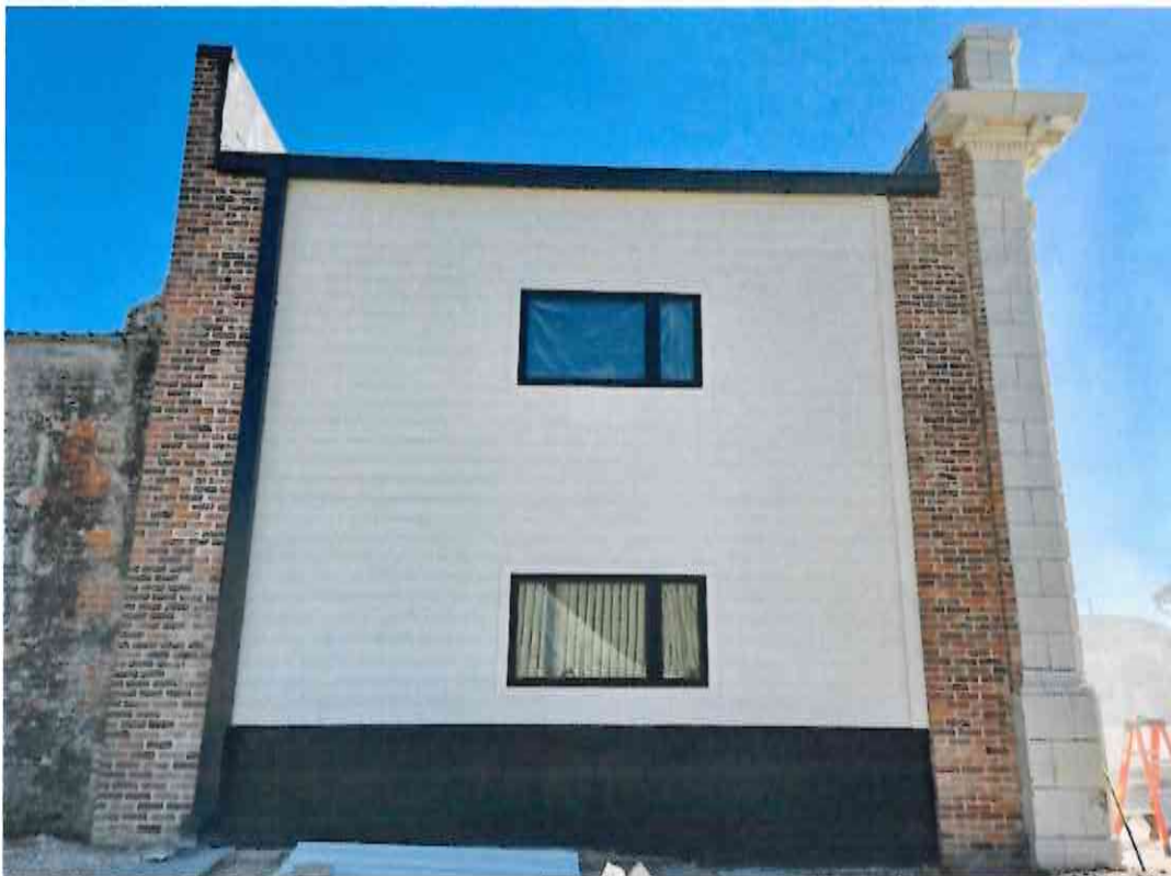
The new rear/north wall.
