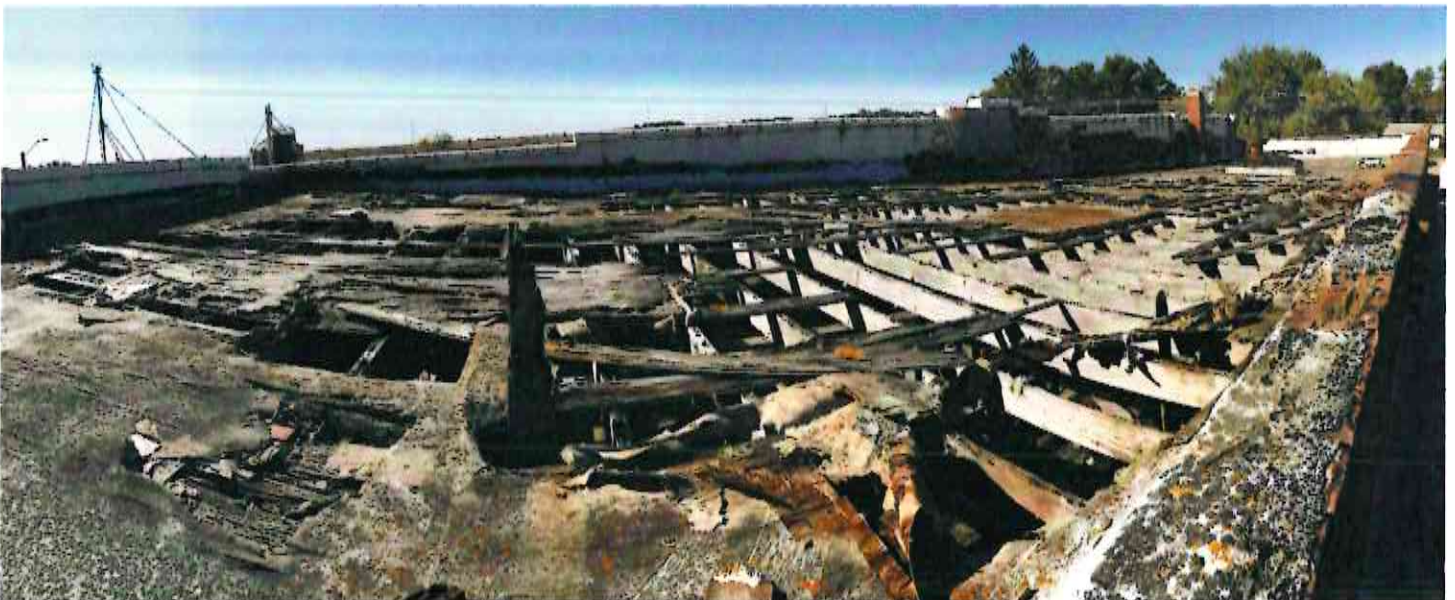
The roof, looking northwest.
